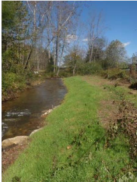
Right channel bank condition after 2015 repairs sta. 1+75 to 2+25 facing upstream, 14 October 2015. No longer considered a problem during MY4 (2015) field surveys.
