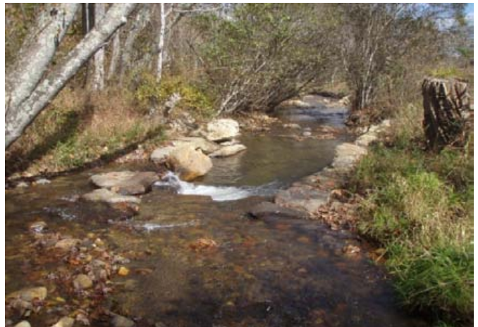
Cross vane, sta. 0+50, facing downstream, 29 October 2013.
