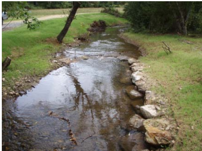
J-hook, sta. 12+75, after construction, facing upstream, 22 Sept 2011.
