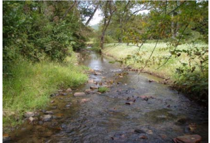
Fence and invasive removal, bank sloping, sta. 5+00, facing downstream, 22 September 2011.
