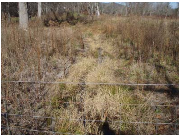
UT2 restored portion, east of Canterfield Lane, 20 November 2012.
