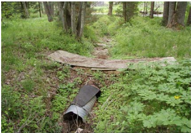
UT1 facing downstream, pre-construction 28 July 2009.
