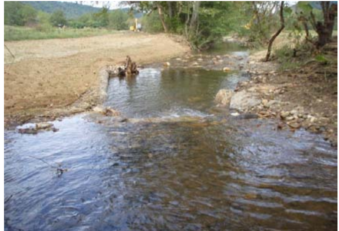
Bank shaping, log vane, and riffle construction, sta. 0+25, 22 September 2011.
