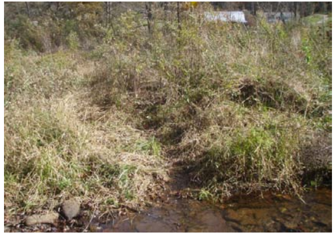
Wetland E reconnected with spring flow from UT2, 29 October 2013.
