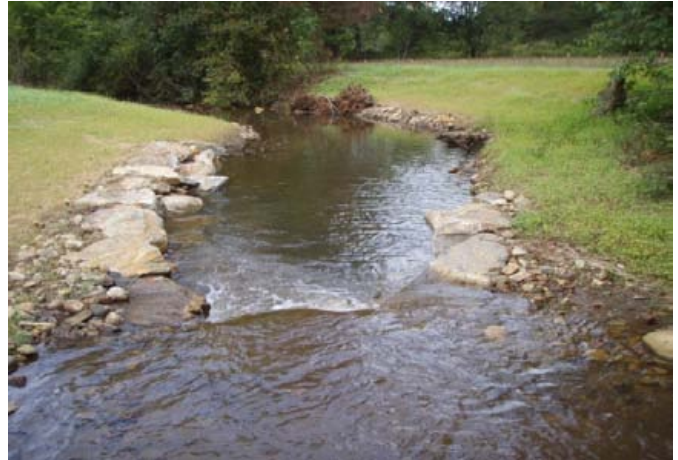
Bank sloping and J-hook, sta. 9+25 to 10+00, 22 September 2011.
