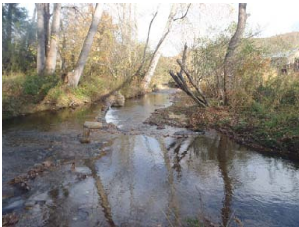
J-hook, sta. 2+50, facing downstream, 12 November 2014.
