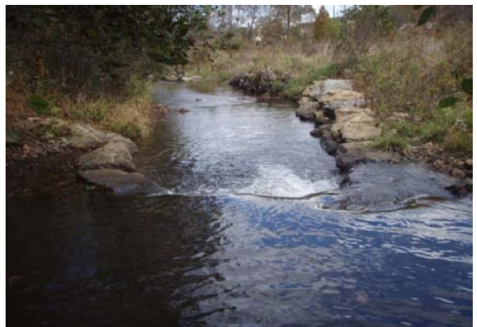
J-hook, sta. 5+00, facing downstream, 29 October 2013.
