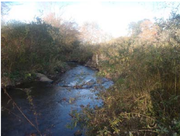
Log vane, root wad, and bank shaping, sta. 7+25 to 8+00, 12 Nov 2014.
