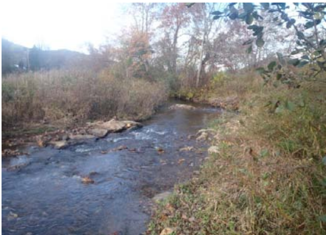
Bank sloping and J-hook, sta. 9+25 to 10+00, 12 Nov 2014.
