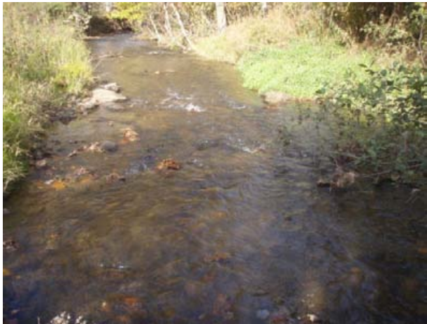
Cross vane, riffle construction, and bank shaping, sta. 6+75, 29 October 2013.
