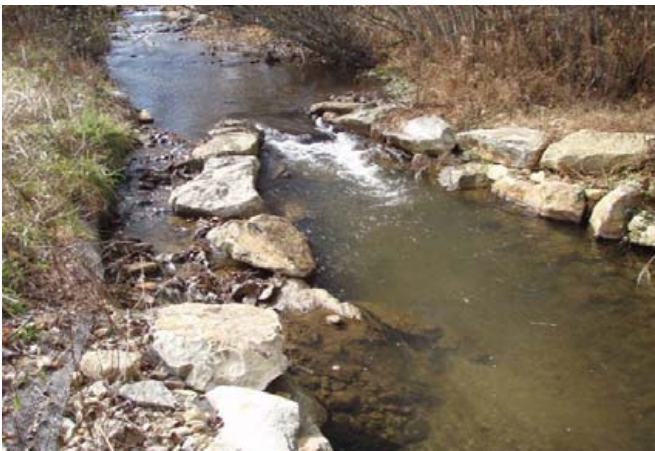
Rock vane, sta. 1+50, facing upstream, 20 November 2012.
