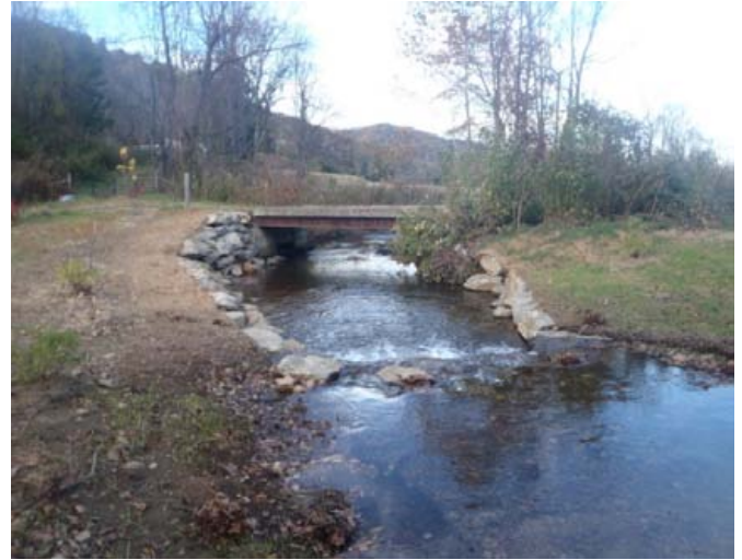
PA-7 station 12+75 facing downstream was repaired and is no longer considered a problem 28 October 2014
