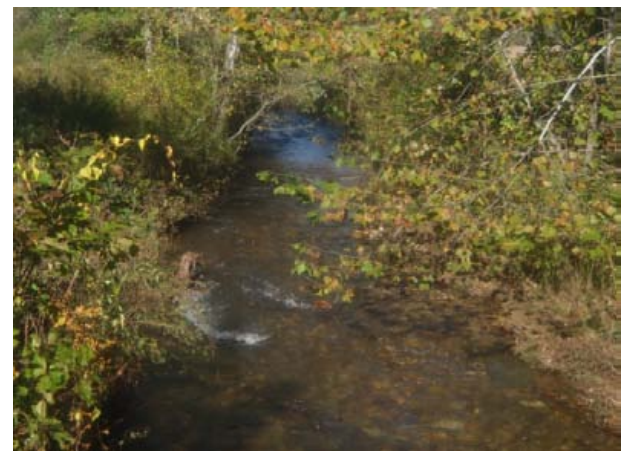
Bank shaping, log vane, and riffle construction, sta. 0+25, 14 October 2015.
