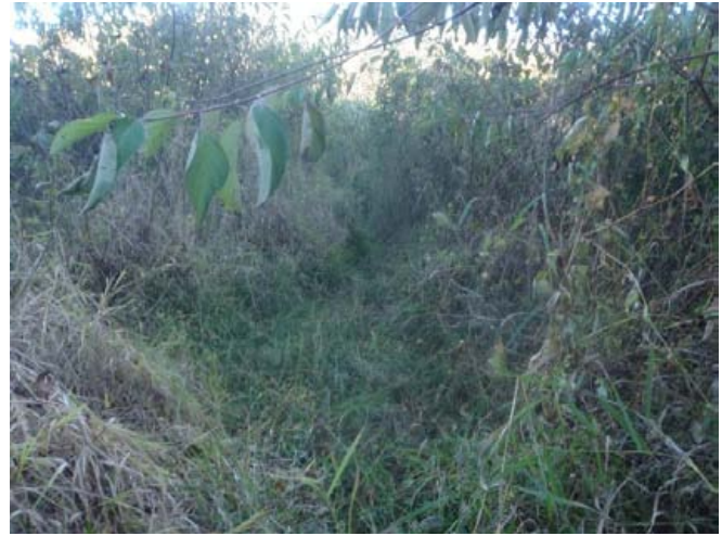
Aggradation due to low flow velocity and dense herbaceous vegetation, sta. 0+00 to 2+00 UT-3 Upper Davis Reach, facing downstream, 15 October 2015.
