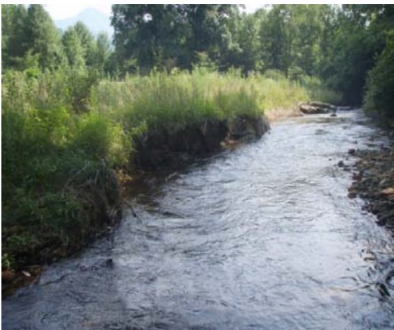
Right channel bank condition after 5 May 2013 flood, sta. 1+75 to 2+25 facing upstream, 18 July 2013.
