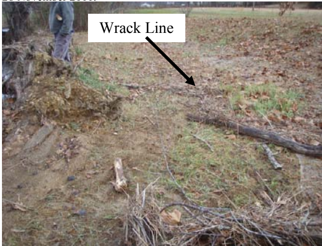
Photo 2 bankfull event on SHC, Roberson property, sta. 8+00 28 November 2011.
