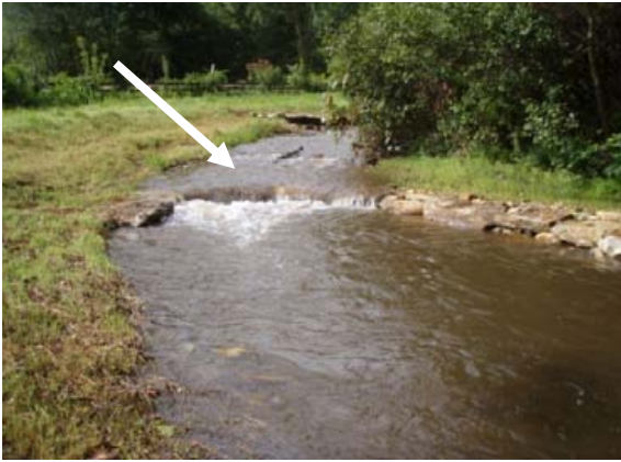
Right channel bank in stable condition, sta. 2+00, facing upstream, 5 September 2011.
