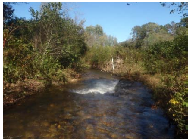
Log vane, root wad, and bank shaping, sta. 7+25 to 8+00, 14 October 2015.
