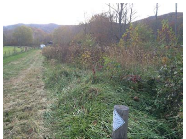
Sta. 6+50 to 8+00, right bank facing upstream, 12 Nov 2014.
