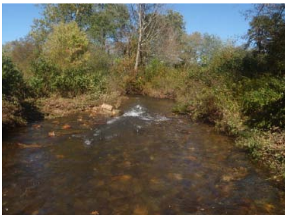
Aggradation and bar formation below J-hook, sta. 9+25 to 9+50, following 5 May 2013 flood event, facing downstream, 14 October 2015.
