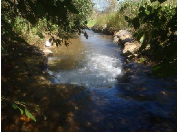
Repaired rock vane, sta 1+50 facing downstream 14 October 2015 No longer considered a problem during MY4 (2015) field surveys.
