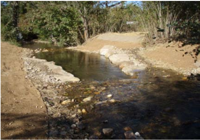
Cross vane, riffle construction, and bank shaping, sta. 6+75, 4 October 2011.
