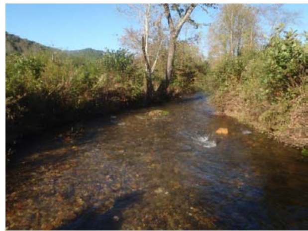
Log vane, root wads, and bank shaping, sta. 2+25 to 3+50, facing downstream, 14 October 2015.
