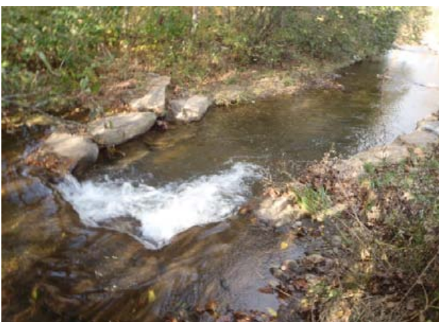
J-hook, sta. 5+00, facing downstream, 12 November 2014.
