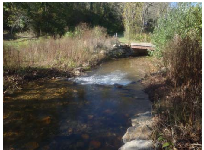
Repaired J-hook, sta. 12+75, facing upstream, 14 October 2015
