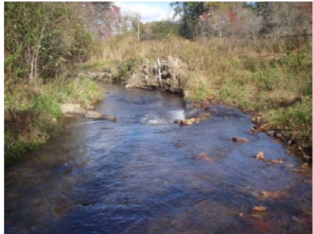
Log vane, root wad, and bank shaping, sta. 7+25 to 8+00, 29 October 2013.
