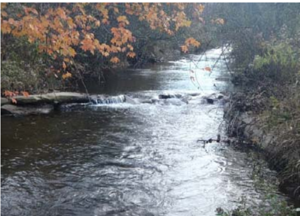
Log vane, root wads, and bank shaping, sta. 4+50, facing upstream 12 Nov 2014.
