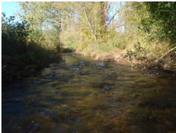
Cross vane, riffle construction, and bank shaping, sta 6+75 14 October 2015
