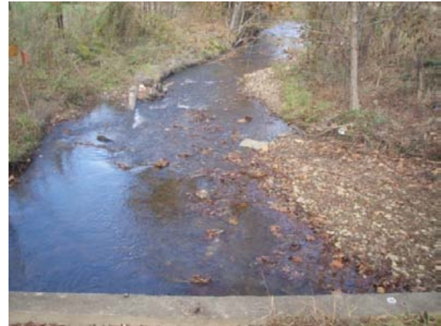
Bank shaping, log vane, and riffle construction, sta. 0+25, 29 October 2013.
