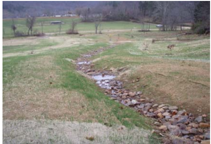
UT3 below ford, Priority I channel restoration, facing downstream, sta. 0+00, 15 November 2011.
