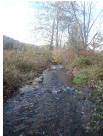
Cross vane, riffle construction, and bank shaping, sta. 6+75, 12 Nov 2014.
