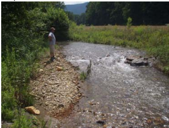
Inner berm formation below J-hook, sta. 9+25 to 9+50, following 5 May 2013 flood event, facing upstream, 18 July 2013.
