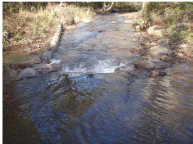
Log vane sta. 1+50 to 2+50, facing downstream, 29 October 2013.
