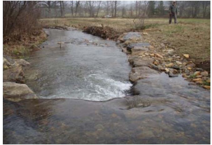
J-hook, sta. 5+00, facing downstream, 5 December 2011.
