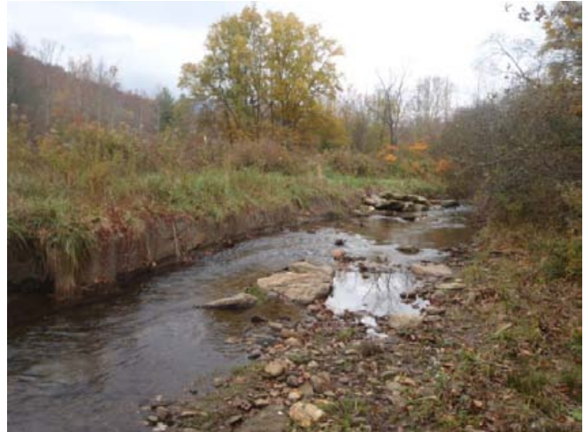
Right channel bank condition sta. 1+45 to 2+75, facing upstream, 28 October 2014.
