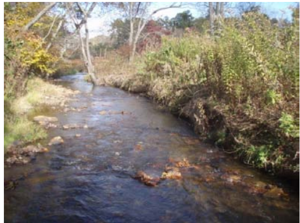
Fence and invasive removal, bank sloping, sta. 5+00, facing downstream, 29 October 2013.
