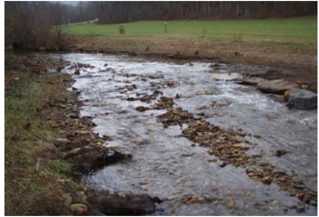
Aggradation and bar formation below J-hook, sta. 9+25 to 9+50, after flood event, facing upstream, 5 December 2011.
