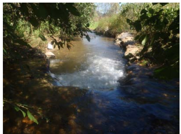
J-hook, sta. 5+00, facing downstream, 14 October 2015.
