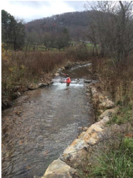
Repaired J-hook, sta. 12+75, facing upstream, 15 October 2015
