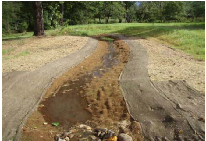
UT2 restored portion, east of Canterfield Lane, 5 September 2011.
