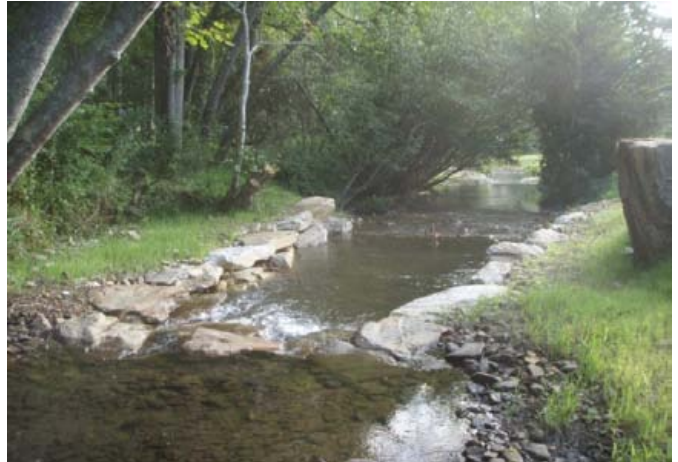
Cross vane, sta. 0+50, facing downstream, 14 August 2011.
