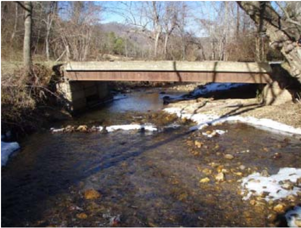
Driveway bridge at lower end of Bura/Roberson properties, sta. 12+50, facing downstream, 22 January 2009.
