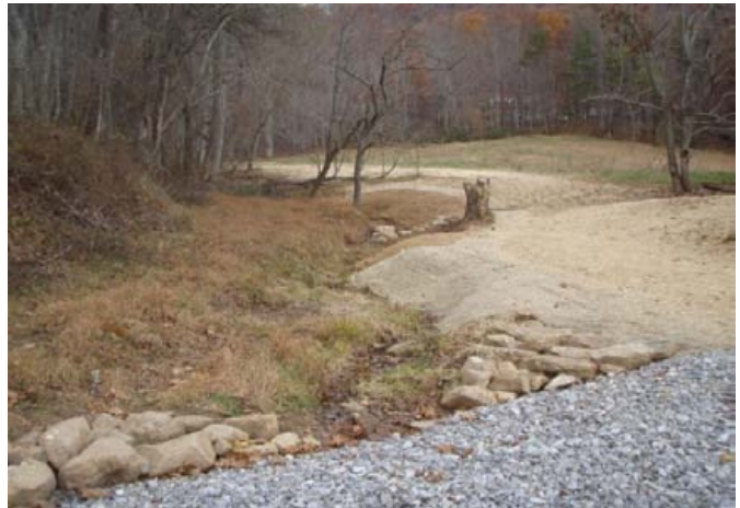
UT3 above ford, invasive removal, cattle exclusion, and bank shaping, facing upstream, 9 November 2011.
