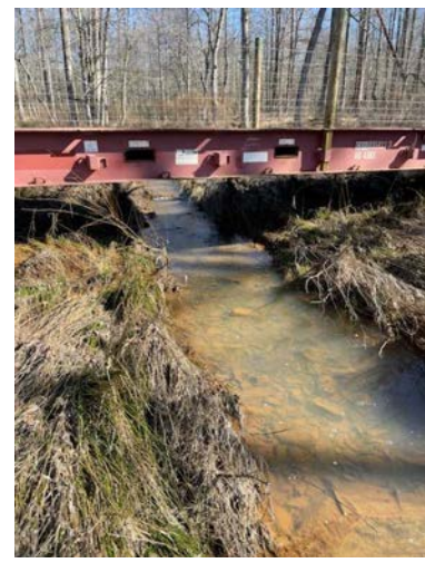
PP-32: Begin Reach 1B, Upstream, Station 33+90 at Crossing. January 29, 2024
