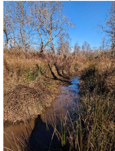
Mid-Channel Bar Repair on Reach 1A (Photo taken December 6, 2023)
