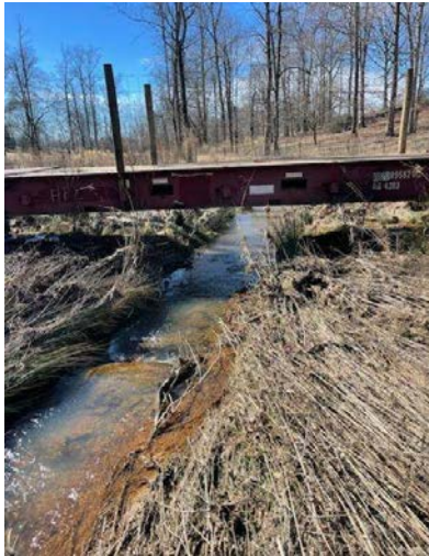
PP-31: End of Reach 1A, Downstream, Station 33+55 at Crossing. January 29, 2024
