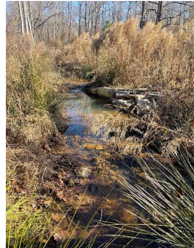
PP-44: Reach 1B, Upstream, Station 41+20. December 6, 2023.
