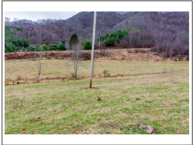
Upper UT3, straight channel in field (Dec. 2019)
