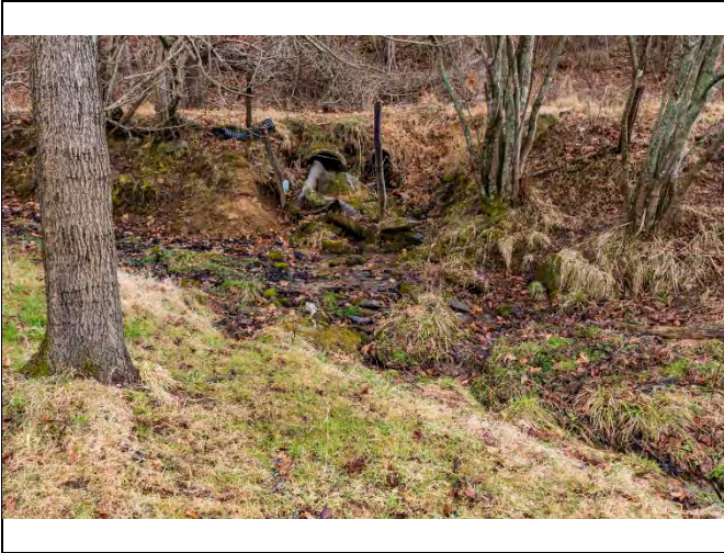
UT1-R3, old culvert (Jan. 2020)
