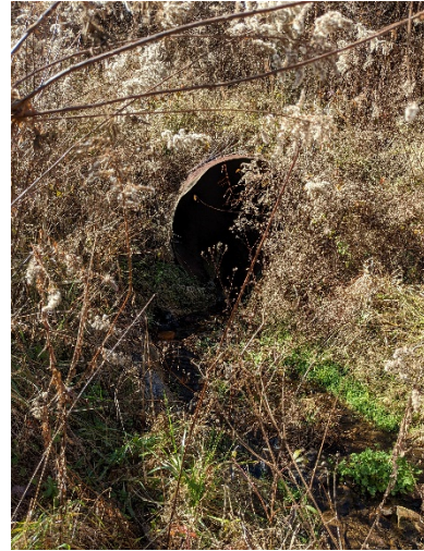
PP-28: UT1, R 4, Station 27+90. Downstream. November 29, 2022
