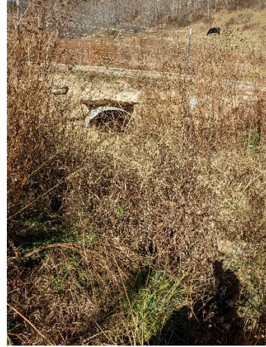
PP-44: UT3, Station 23+15. Upstream. November 9, 2022
