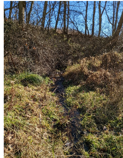
PP-58: UT1, R 4, Station 37+60. Downstream. End of Project. November 29, 2022
