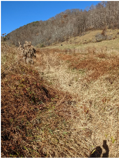
PP-39: UT3, Station 18+75. Upstream. November 9, 2022
