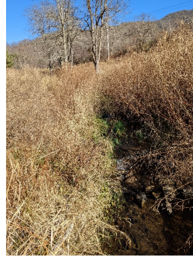
PP-50: UT1, R 4, Station 32+50. Upstream. November 29, 2022
