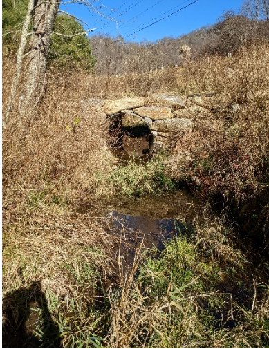
PP-49: UT1, R 4, Station 31+20. Upstream. November 29, 2022
