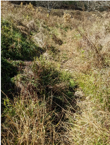
PP-31: UT3, Station 11+10. Upstream. November 9, 2022
