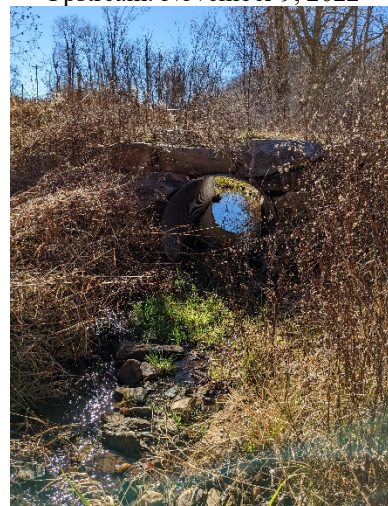
PP-48: UT1, R 4, Station 30+50. Downstream. November 29, 2022
