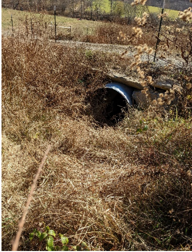
PP-43: UT3, Station 22+15. Downstream. November 9, 2022
