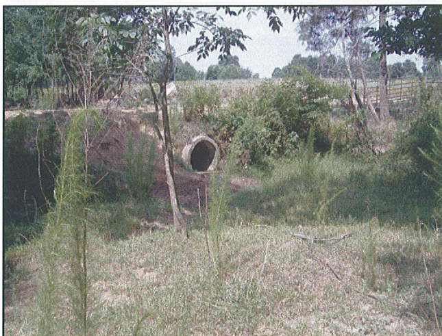
Photo 9. Facing west at the existing pipe that underlies the stream crossing.
