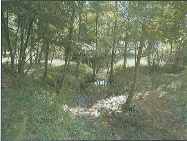
Photo 13. Facing southwest (downstream) along the UT Altamahaw Creek Stream Segment #1 towards the existing culvert.
