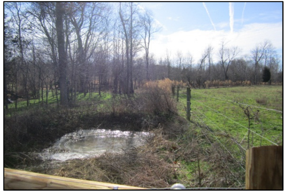
Photostation 8. Facing southwest from corner at existing west corner of crossing.
