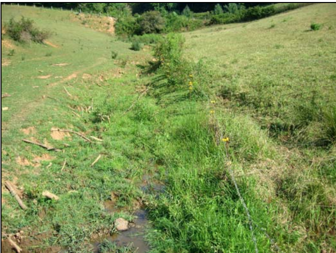
Mainstem looking upstream toward Wetland 4 and the dam.
