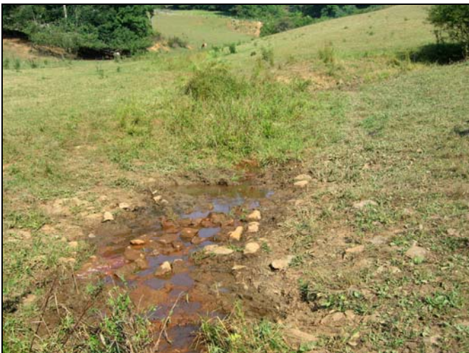
Looking upstream from cattle crossing to the confluence of Tributary 2 and the Mainstem.
