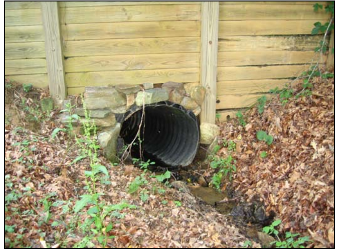
Culvert carrying Tributary 2 beneath driveway.
