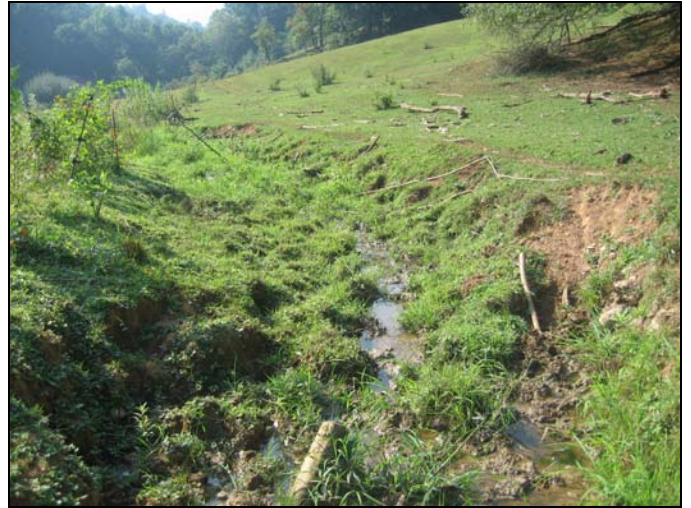
Impaired portion of the Mainstem.
