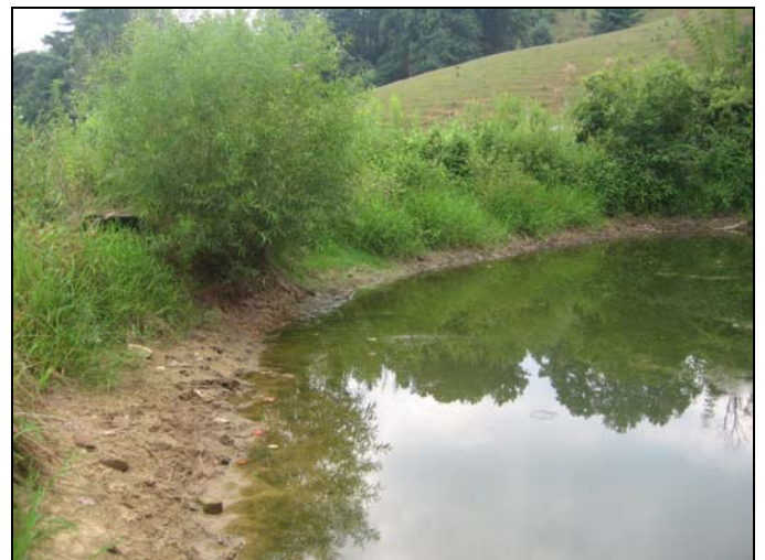
The Mainstem flows through another impoundment, Wetland 1A. Looking downstream at the dam.
