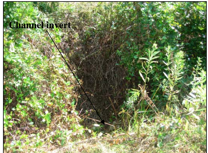
The incised channel at a swath cut through the dense invasive vegetation.
