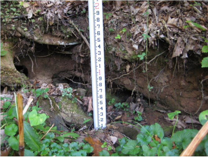
Mainstem Reach B – steep and eroding left bank.
