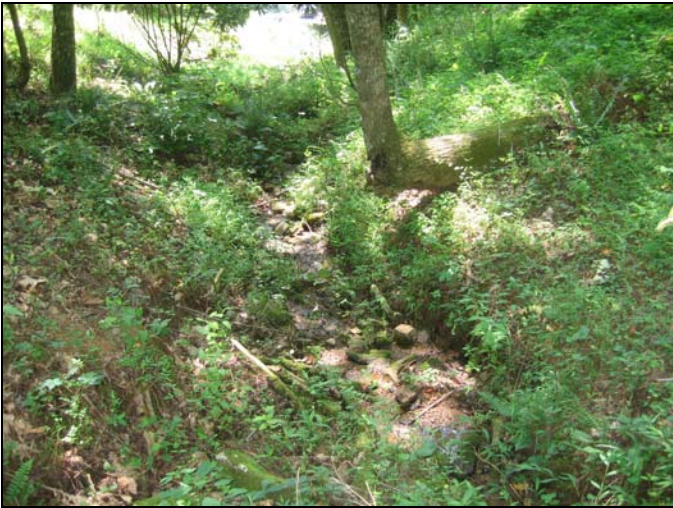
Stable portion of Tributary 2 in the upper Project Reach.
