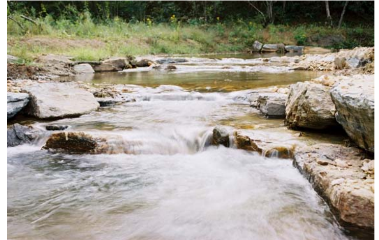
Double Drop Rock Cross Vane
