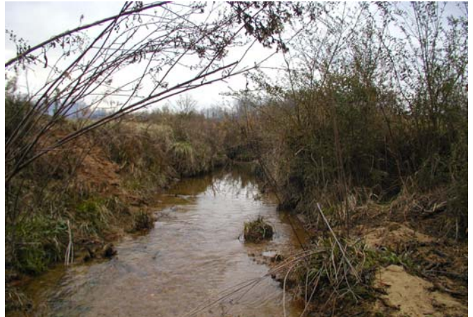
Localized stream overwidening on the Hurley property
