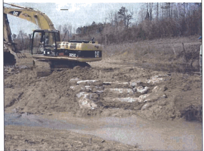
Step Pool Station 34+00
