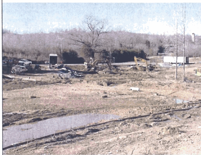
Site Picture Looking Downstream
