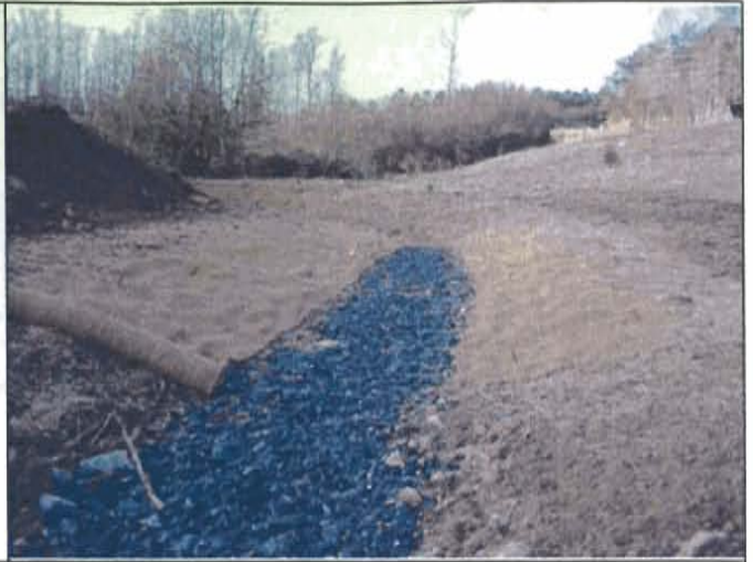
Constructed Riffle during Construction
