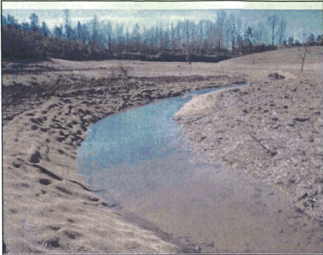
Station 17+40 Pool Construction
