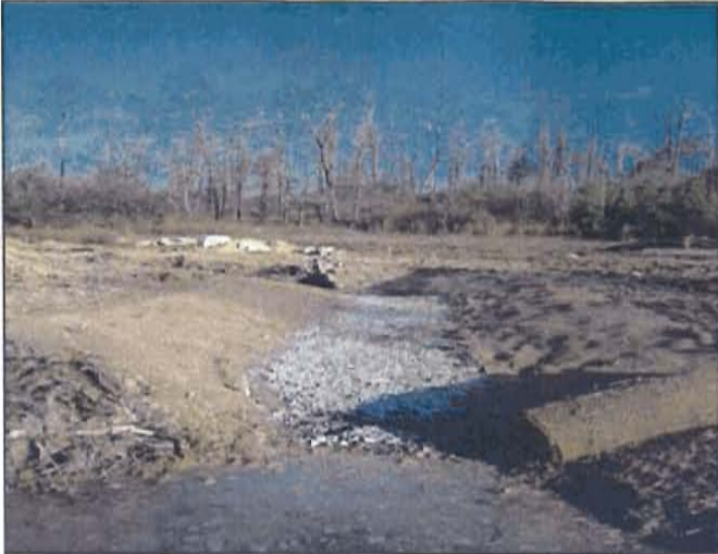
Station 12+50 Riffle construction
