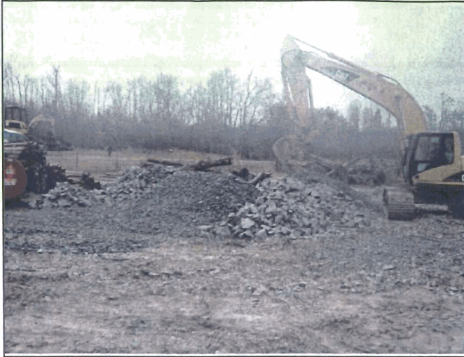
Stock Piling Material for Construction
