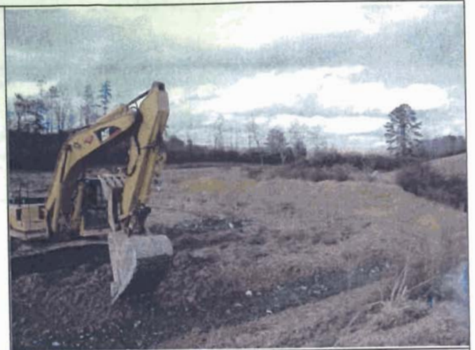
Construction of Riffle Station 26+25
