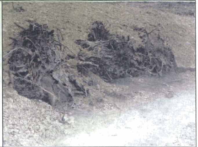
Root Wad Installation during Construction
