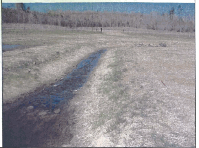
As-Built Typical Constructed Riffle
