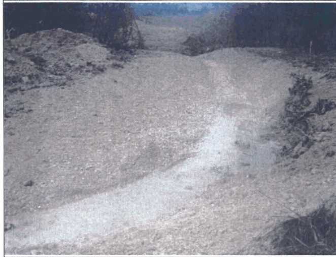
Station 14+00 Riffle Construction
