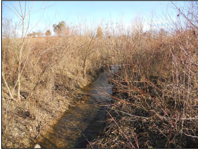
M-29 View Upstream Main Channel (2/2011)
