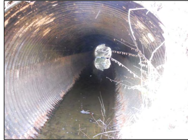
M-1 View Downstream Main Channel (2/2011)
