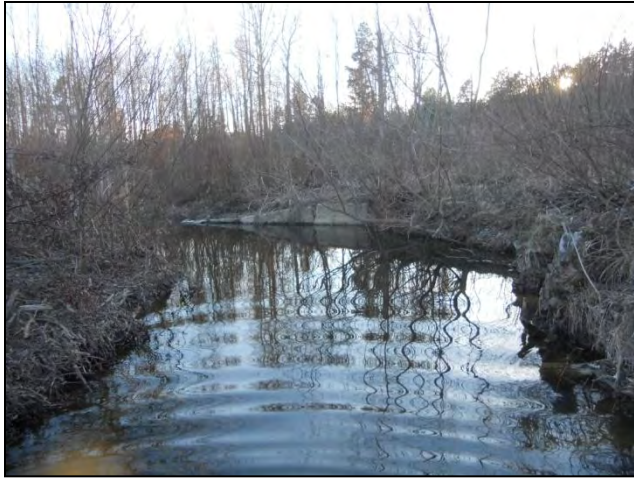
M-58 View Upstream Main Channel (2/2011)
