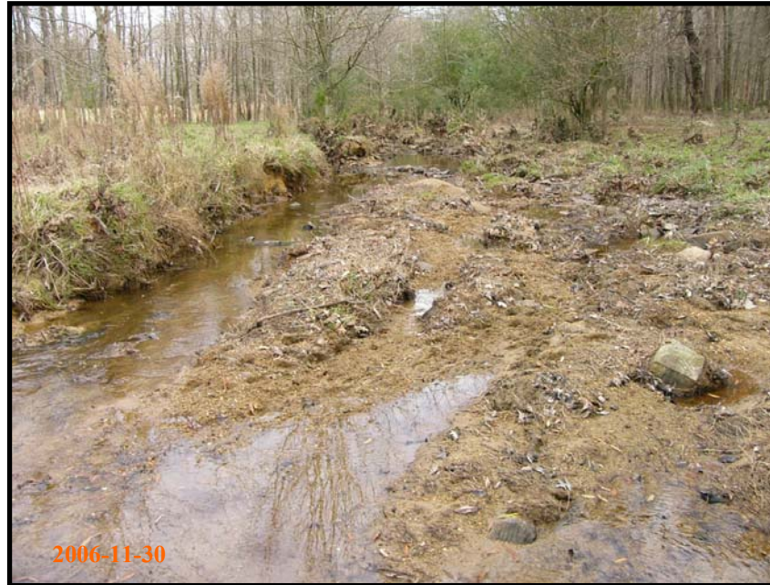
Northern UT looking downstream at cattle access point, and channel over widening. Notice aggradation where channel has over widened.
