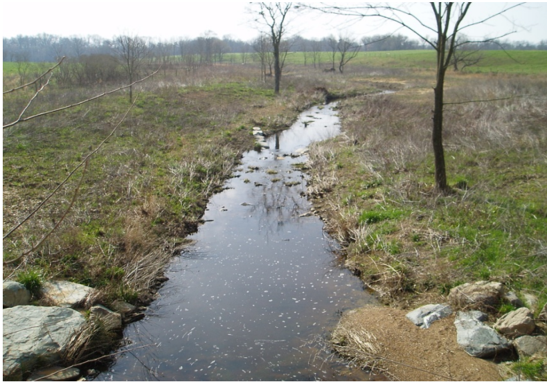
PP 1 Looking at northern UT from NC 902 (Sta. 0+0)(3/25/10)
