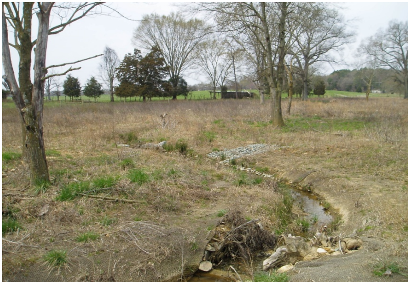
PP 16 Looking downstream on southern UT (Sta. 24+20)(03/25/10)
