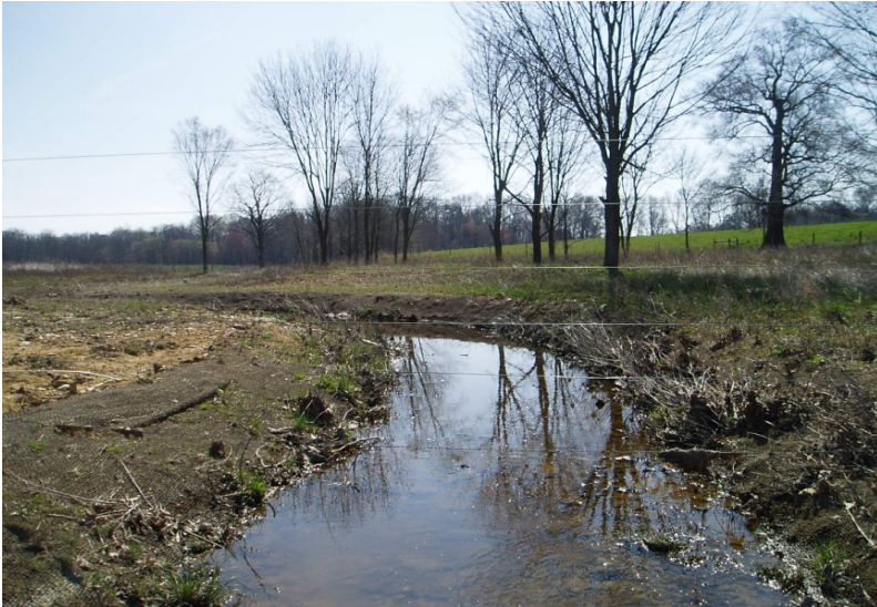
PP 5 At cattle crossing looking downstream (Sta. 19+30)(03/24/10)
