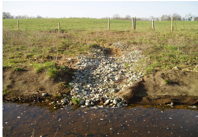
PP 4 Looking at floodplain interceptor on northern UT (Sta. 17+55)(3/24/10)
