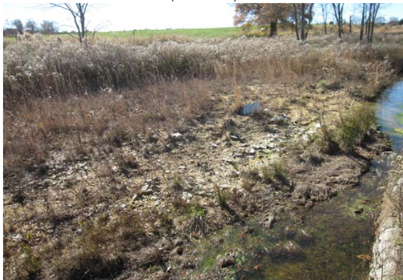
4. Bank scour/bare soil (Sta. 22+70) - Northern UT
