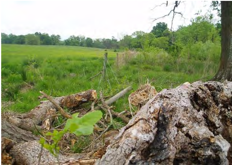
11. S-sta-1750.LB. Apr.2013. Tree fallen on fence
