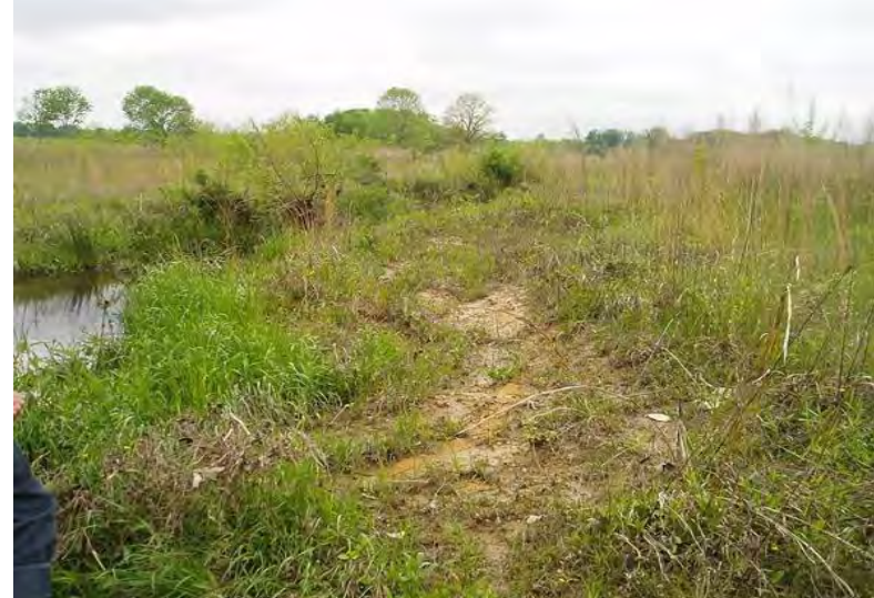
4. N-sta-3700.LB Erosion.Apr 2013. Thin veg cover, no woody.
