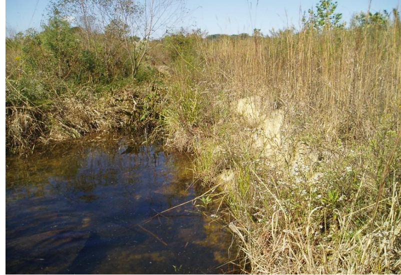
2. N-sta-3450.LB Erosion.Oct 2014. Thin veg cover, no woody.
