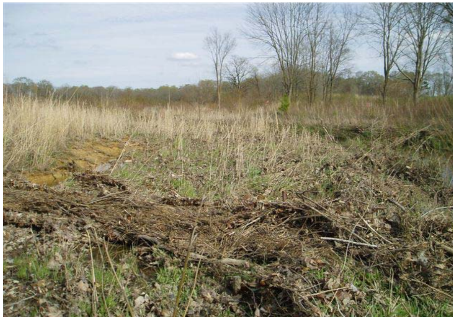
North Trib - Matted vegetation and wrack deposit, Sta 19+50, 08 Apr 2014
