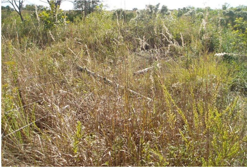
9. N-sta-1930.LB. Oct.2014. Fence collapse at cattle crossing
