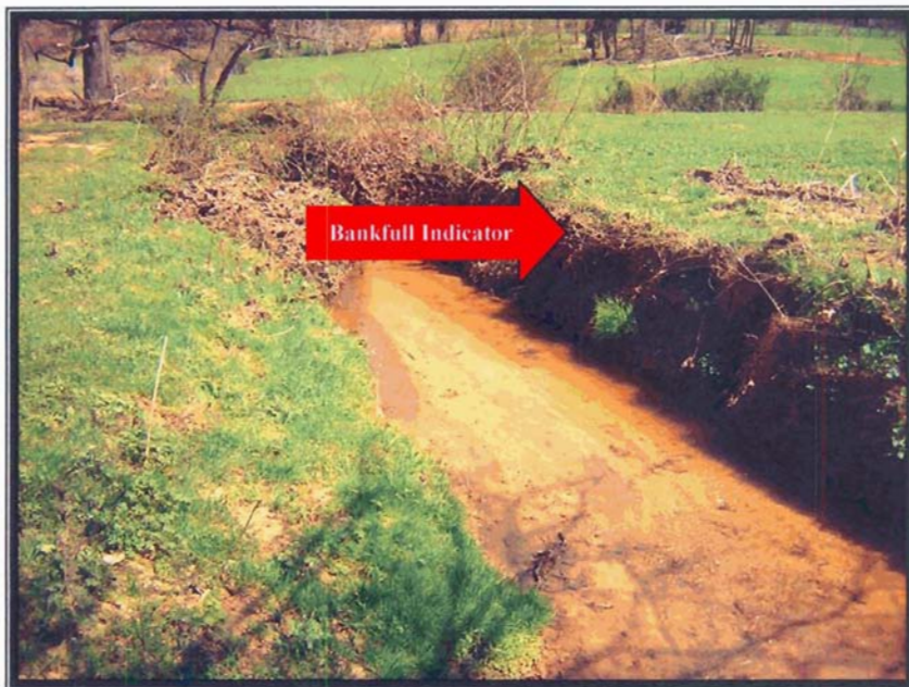
Reach D (Tributary 1) Bankfull Indicator (looking downstream)
