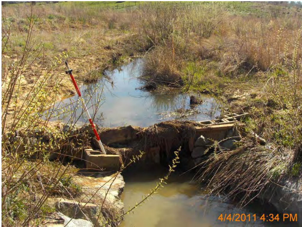
Photo taken from right bank looking upstream
