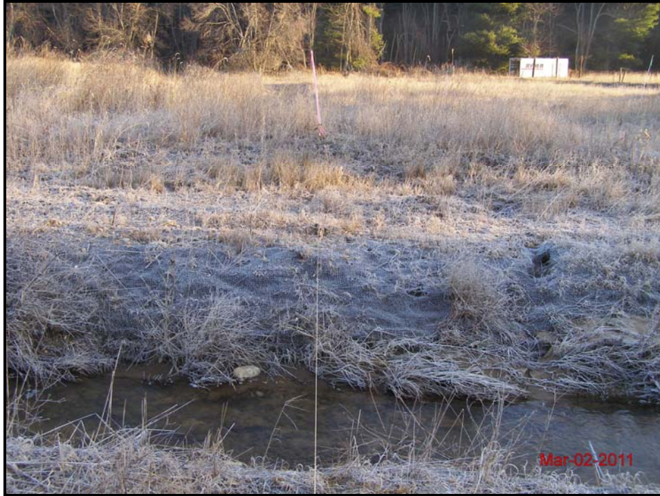
Cross-Section 5 – Riffle (Looking at Left Bank Descending) Monitoring Year 1 – March 2, 2011
