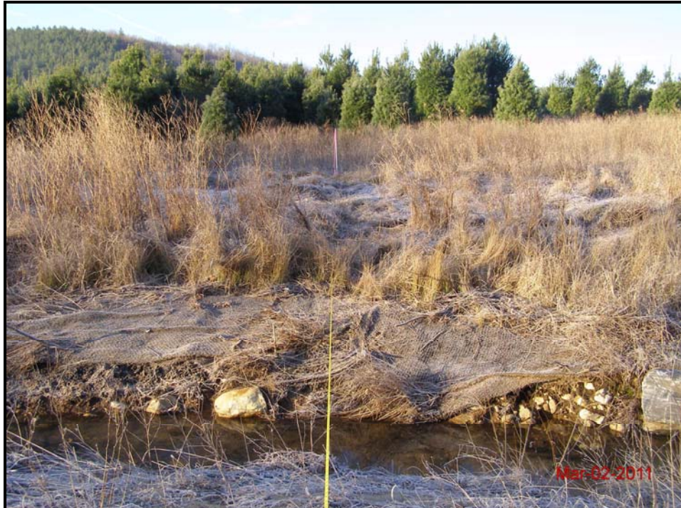
Cross-Section 4 – Pool (Looking at Right Bank Descending) Monitoring Year 1 – March 1, 2011
