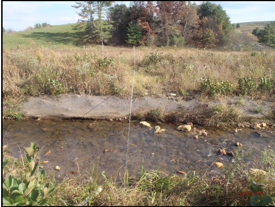
Cross-Section 6 – Riffle (Looking at Left Bank Descending) Monitoring Year 2 – October 17, 2011
