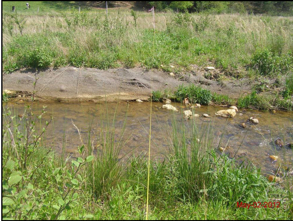
Cross-Section 6 – Riffle Left Bank Descending Monitoring Year 3 – May 2, 2012
