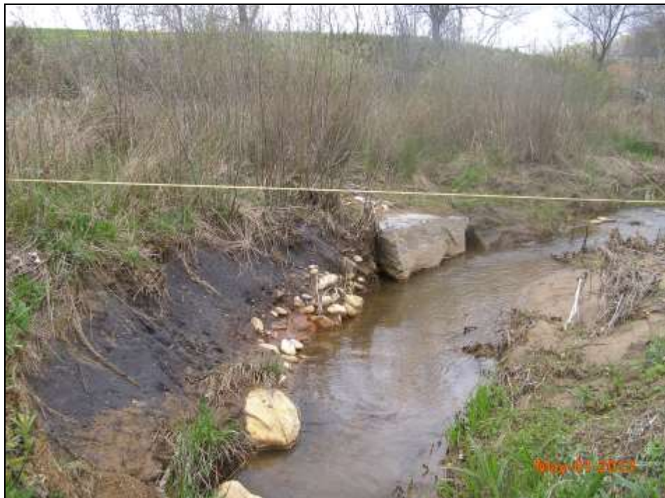
Cross-Section 4 – Pool Upstream Monitoring Year 4 – May 1, 2013
