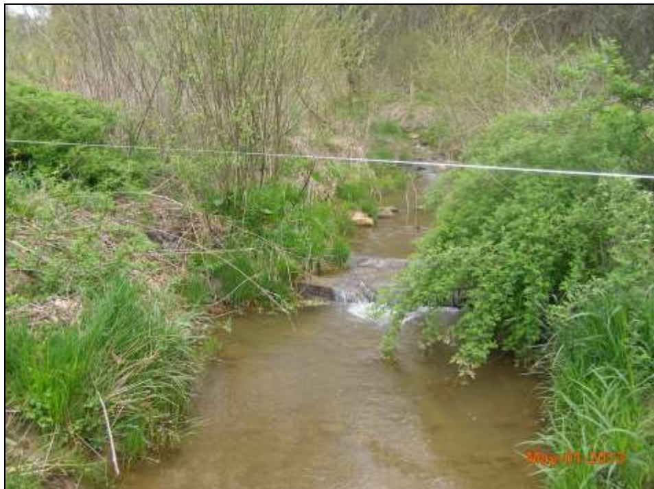
Cross-Section 2 – Pool Upstream Monitoring Year 4 – May 1, 2013
