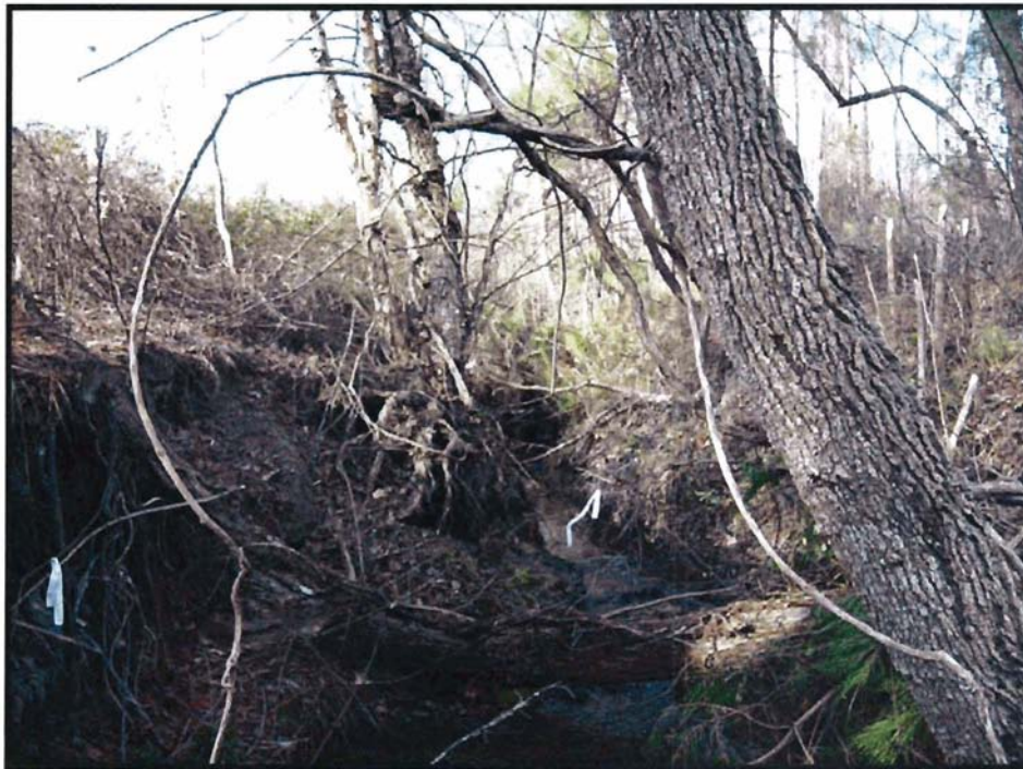
Existing Channel Along Upper Section of Project
