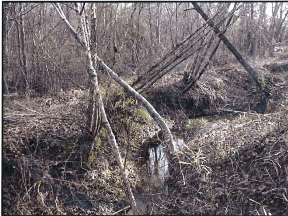
Existing Channel Along Upper Section of Project
