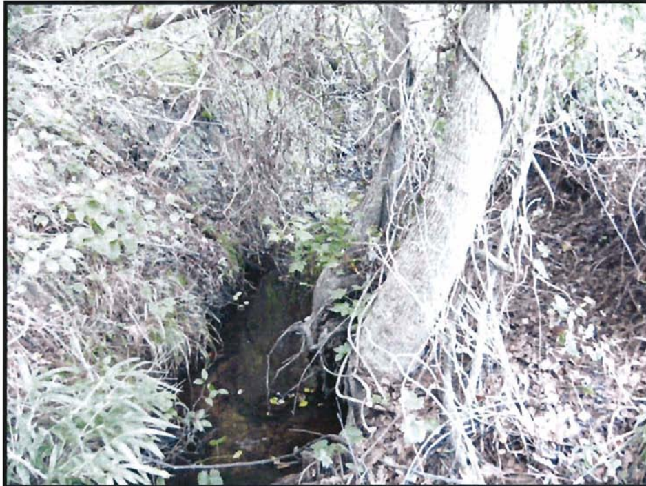
Existing Channel Looking Downstream at the Top of Beaver Dam
