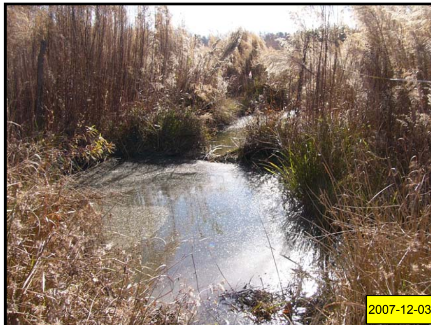
PA – 2 Looking Downstream at Dam
