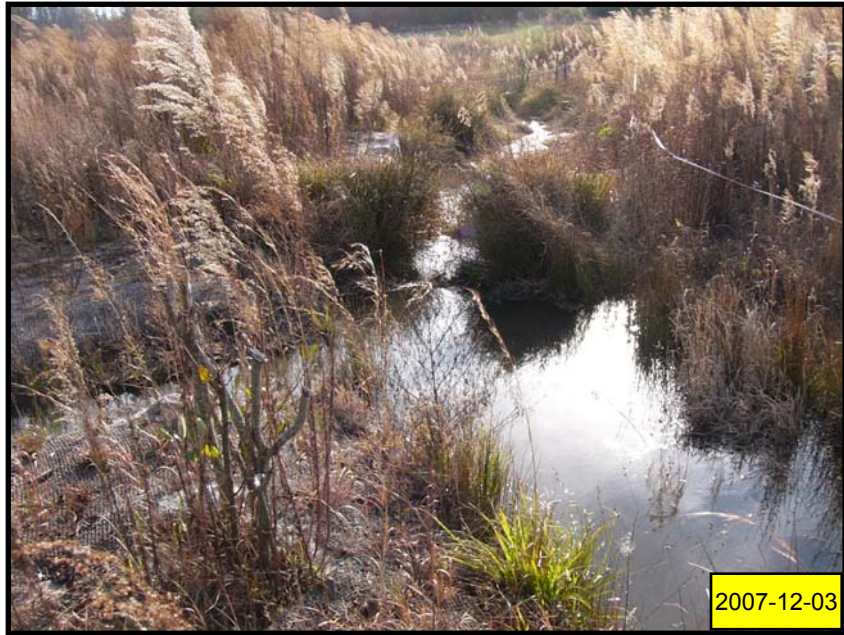
PA – 3 Looking Downstream at Dam
