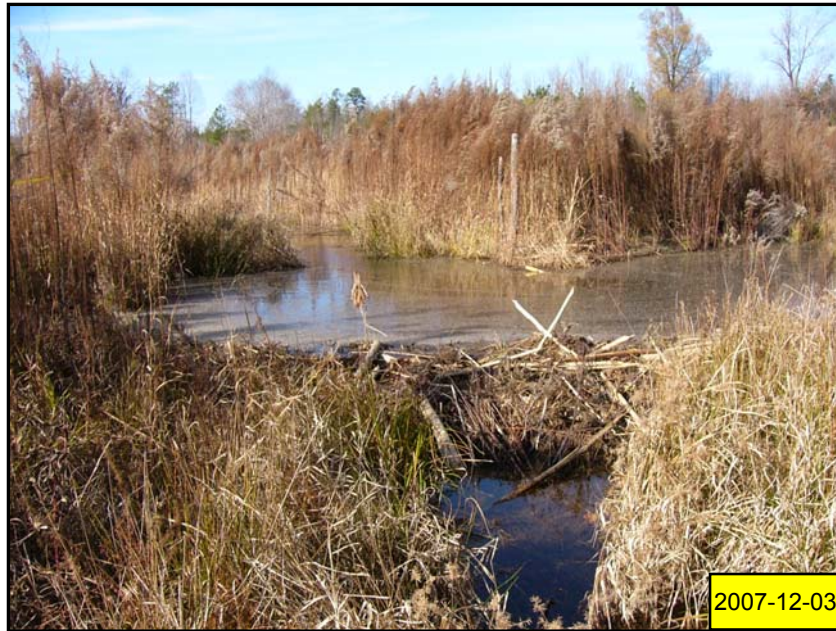
PA – 1 Looking Upstream at Dam
