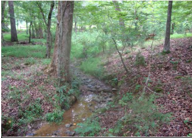
As-Built/Year 1 Survey: August 2012
