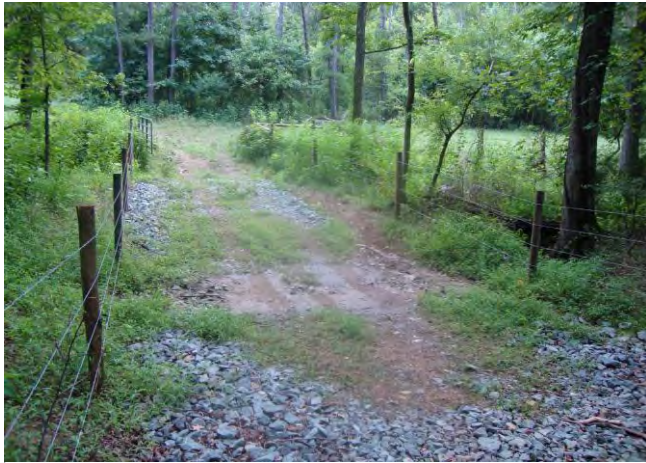
As-Built/Year 1 Survey: August 2012
