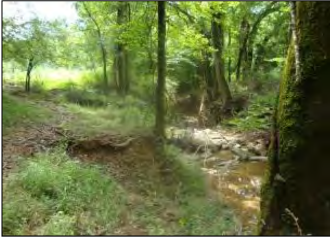
As-Built/Year 1 Survey: August 2012
