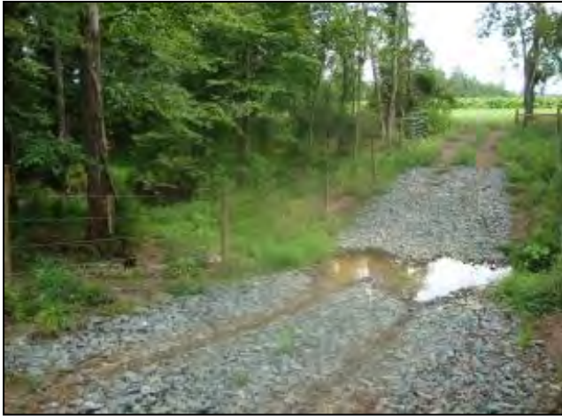
As-Built/Year 1 Survey: August 2012
