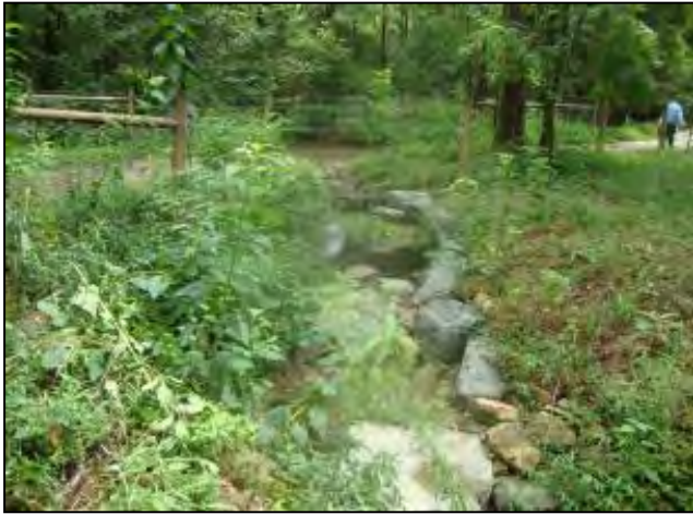
As-Built/Year 1 Survey: August 2012
