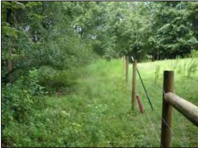
As-Built/Year 1 Survey: August 2012
