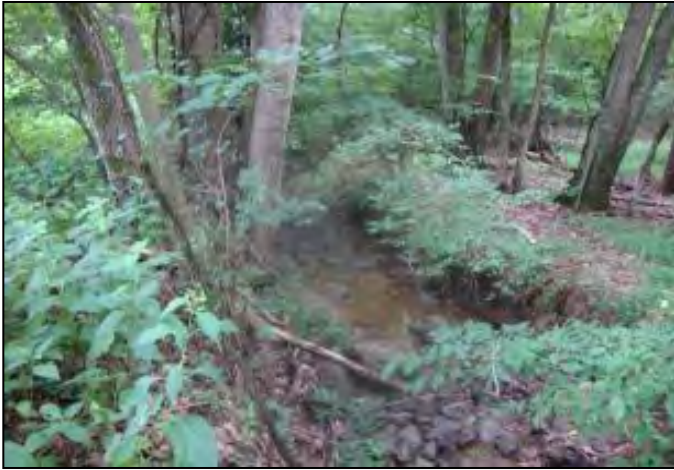
As-Built/Year 1 Survey: August 2012
