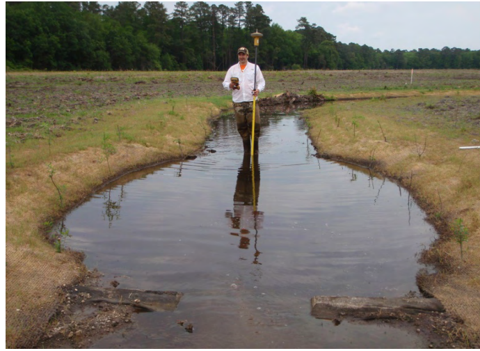
Sta 75+30 Looking Downstream
