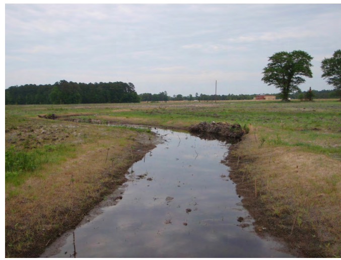
Sta 54+98 Looking Downstream
