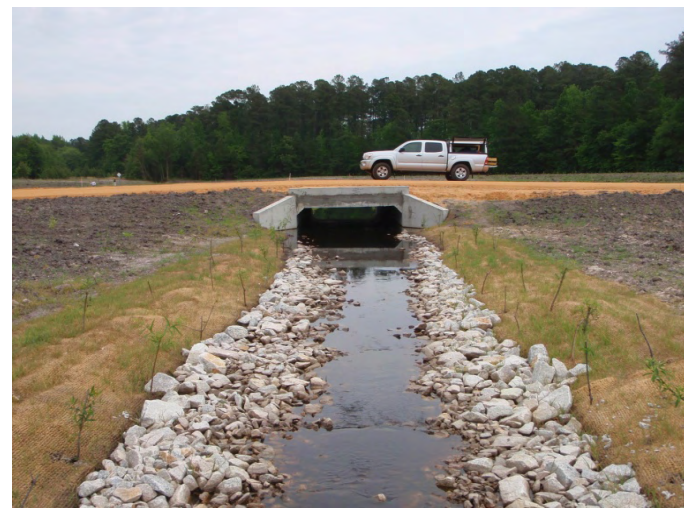
Sta 74+84 Looking Downstream
