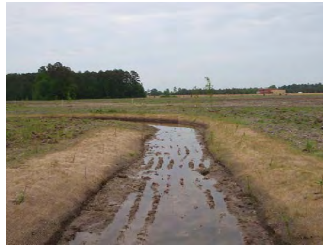
Sta 62+87 Looking Downstream
