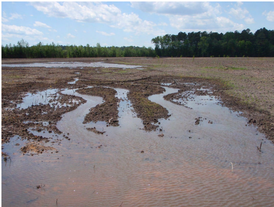
Photo Station S12 – Stream channel looking upstream at upper road crossing (4/26/2010 Year 0)
