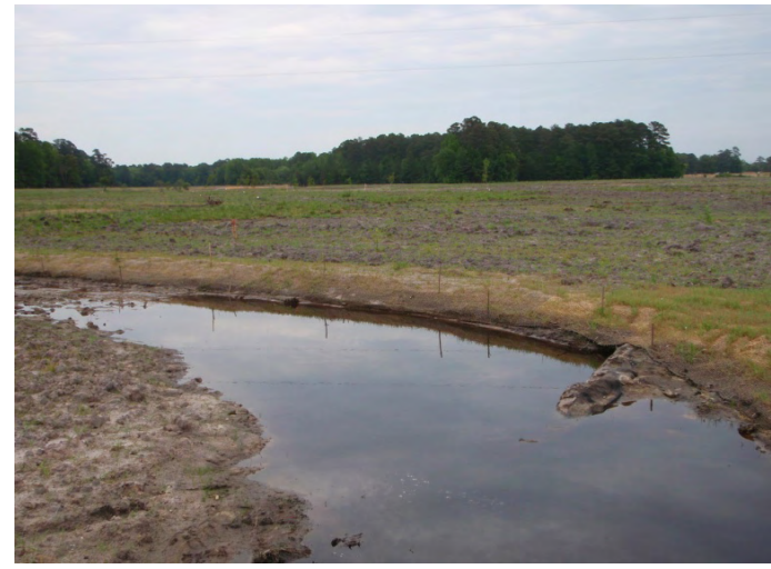
Sta 59+09 Looking Downstream
