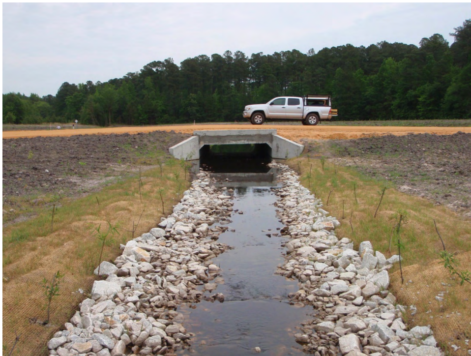
Photo Station S8 – Stream channel looking downstream at cross-section 8 Station 74+84 (5/4/2010 Year 0)
