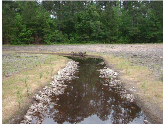
Sta 80+45 Looking Downstream
