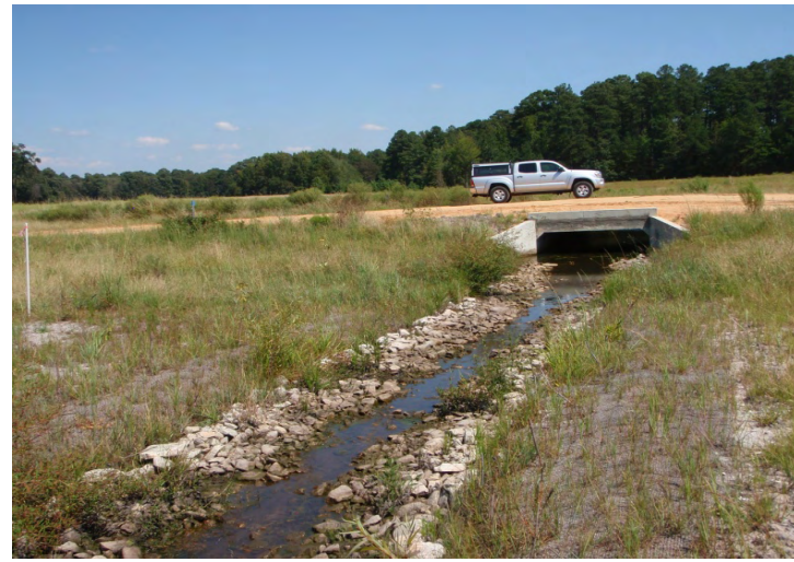
Sta 74+84 Looking Downstream
