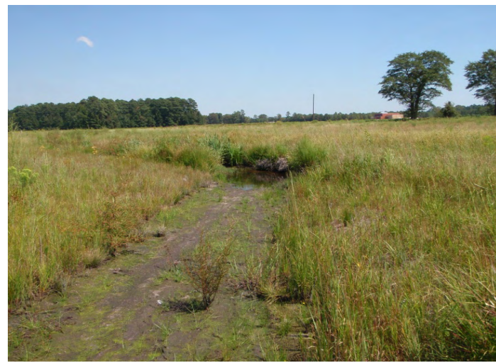
Sta 54+98 Looking Downstream
