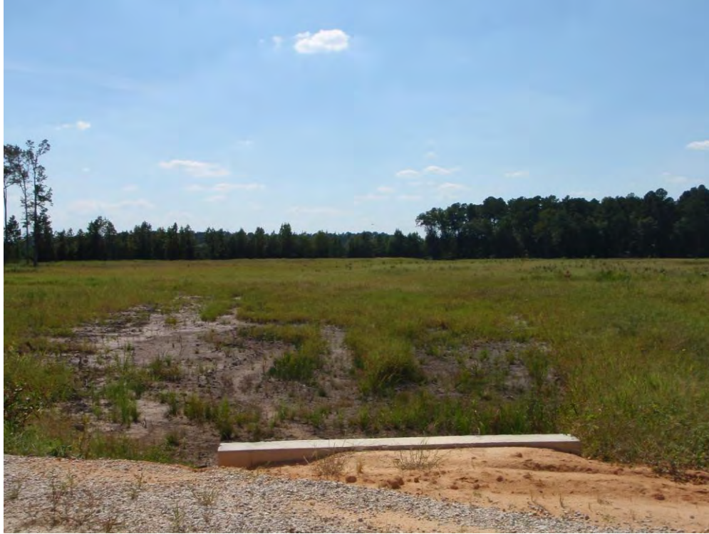
Photo B11 – (Photo Station S12) Stream channel looking upstream at upper road crossing (9/16/2010 Year 1)
