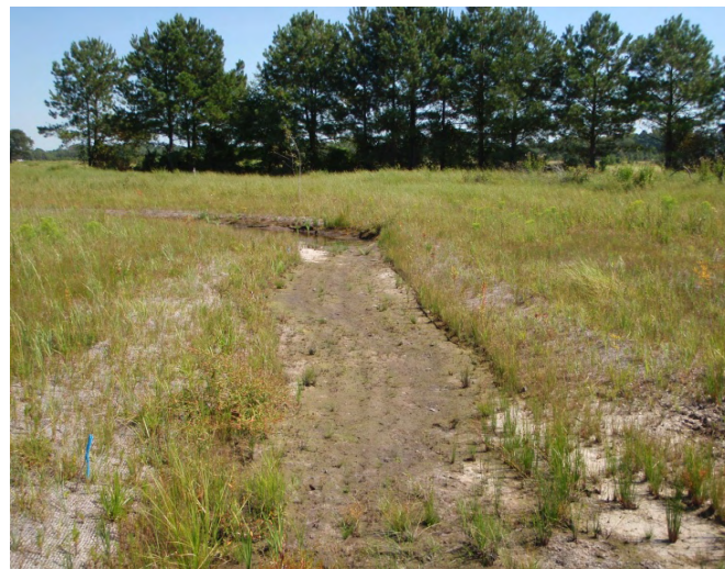
Sta 48+81 Looking Downstream
