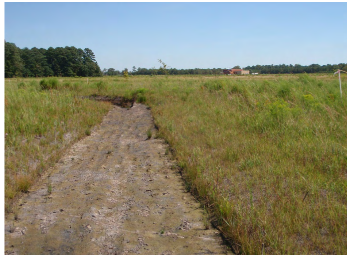
Sta 62+87 Looking Downstream
