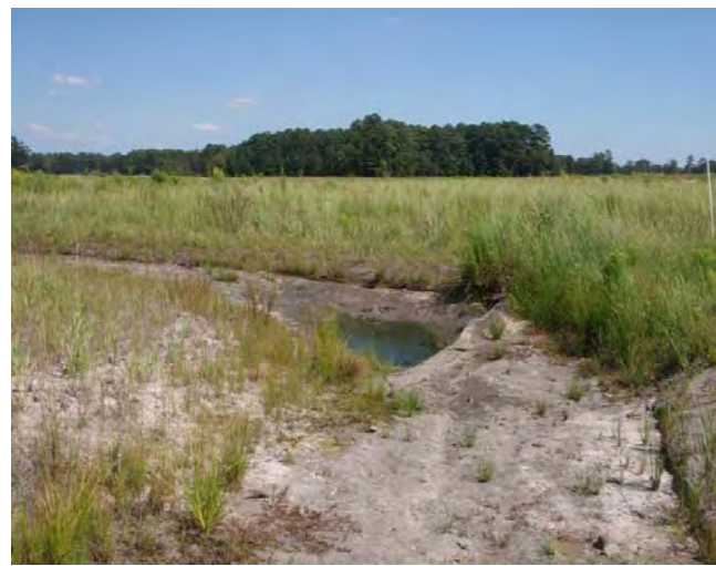
Sta 59+09 Looking Downstream
