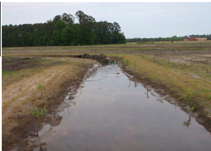
Sta 68+24 Looking Downstream
