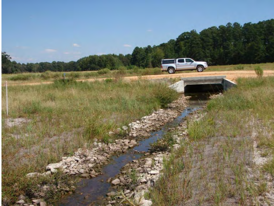
Photo B7 – (Photo Station S8) Cross-section 8 looking downstream at Station 74+84 (9/16/2010 Year 1)
