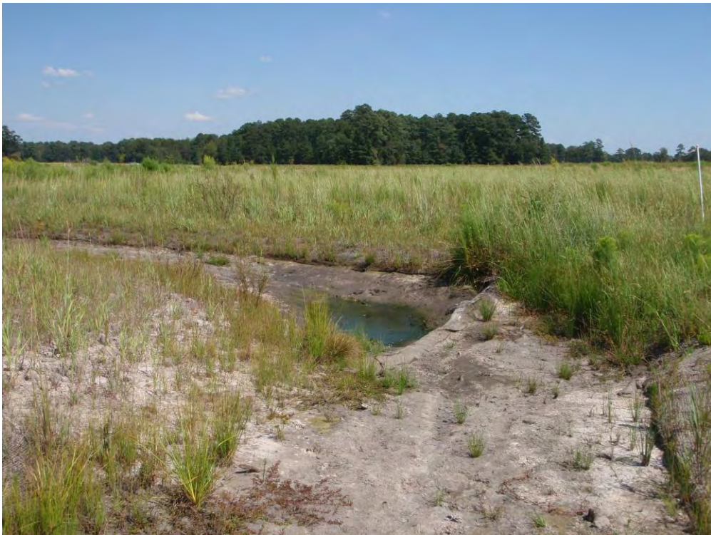
Photo B4 – (Photo Station S4) Cross-section 4 looking downstream at Station 59+09 (9/16/2010 Year 1)
