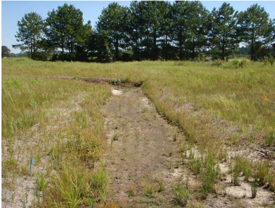
Photo B1 – (Photo Station 1) Cross-section 1 looking downstream at Station 48+81 (9/16/2010 Year 1)
