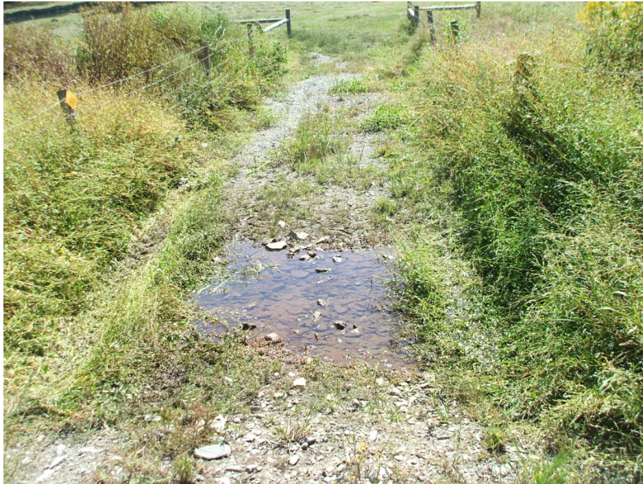
Main Reach Station 10+50 – Stream Crossing
