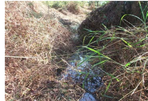
Photo of Cross-Section 12 - Looking Downstream
