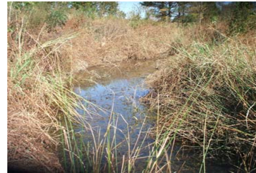
Photo of Cross-Section 10 - Looking Downstream
