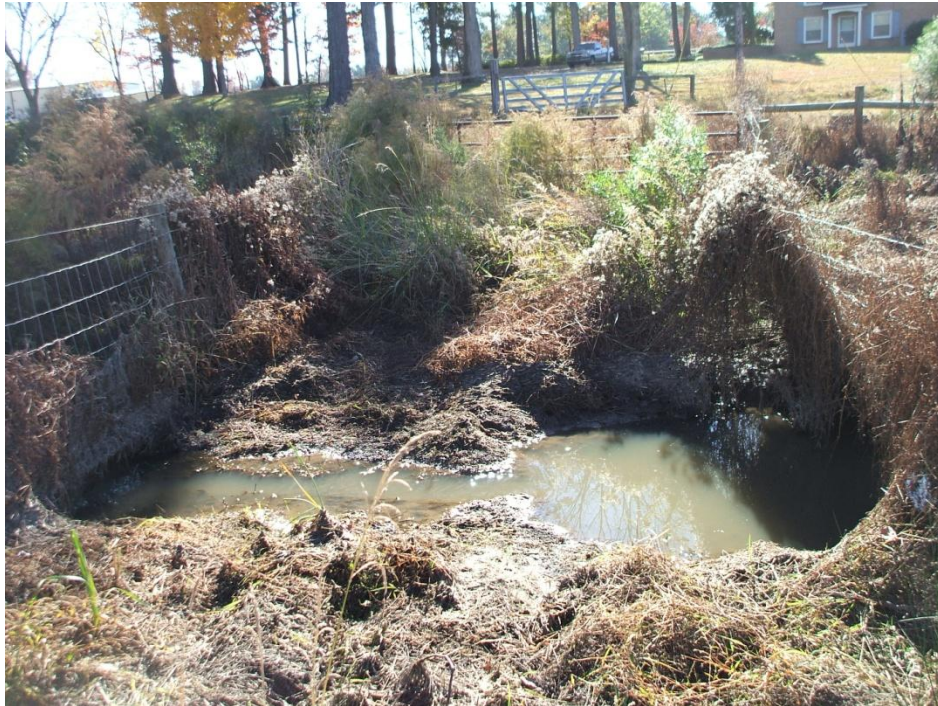
6 - Main Reach Station 10+50 – Stream Crossing
