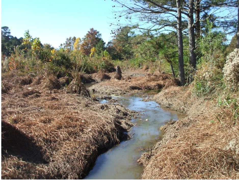
3 - Main Reach Station 6+50 – Looking upstream
