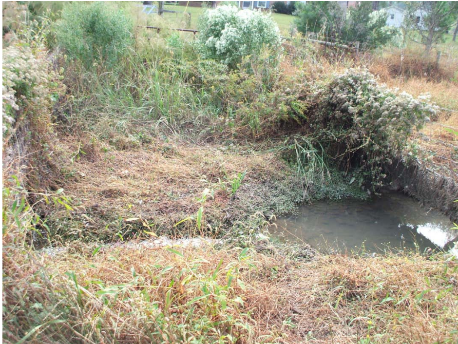
6 - Main Reach Station 10+50 – Stream Crossing
