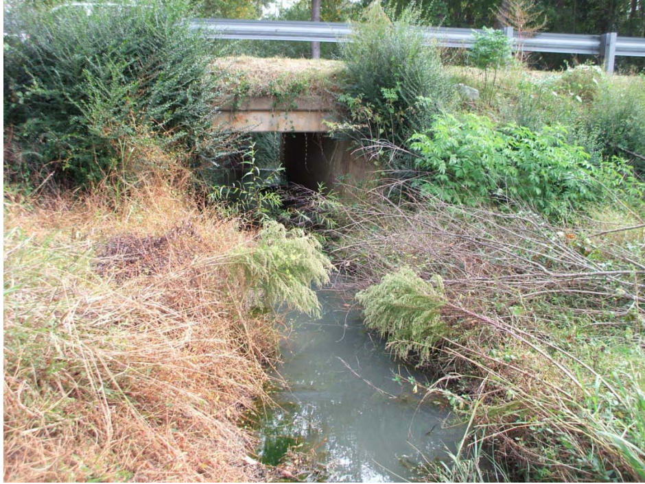
9 - Main Reach Station 12+50 – Looking downstream (End of Main Reach)
