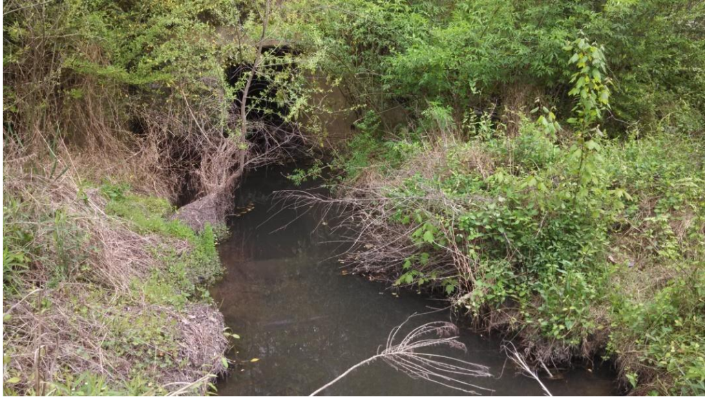
9 - Main Reach Station 12+50 – Looking downstream (End of Main Reach)
