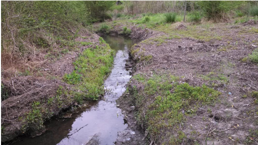
4 - Main Reach Station 6+50 – Looking downstream
