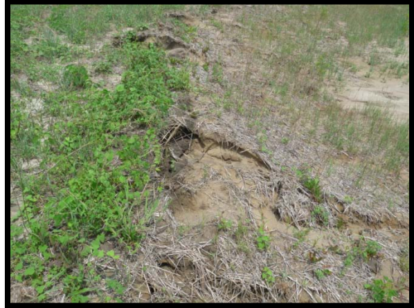
3.18 Poor vegetation growth on terrace slope
