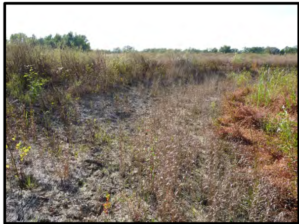
3.20 Minor wash on terrace slope
