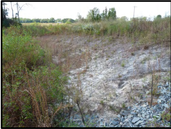
3.17 Sparse vegetation on terrace slope
