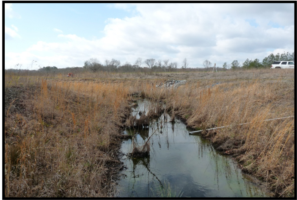
XS 11, Sta. 39+19, Looking Downstream
