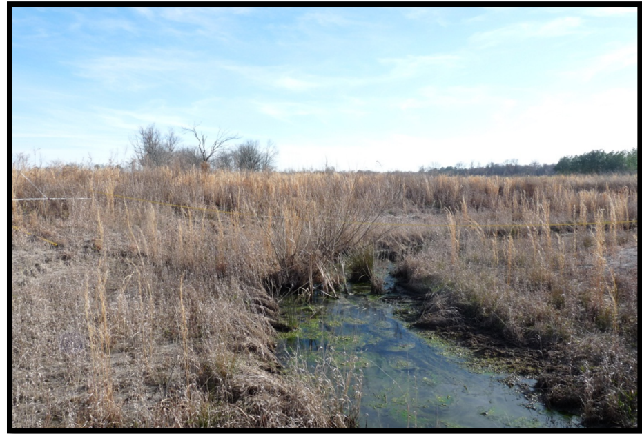
XS 8, Sta. 30+98, Looking Downstream
