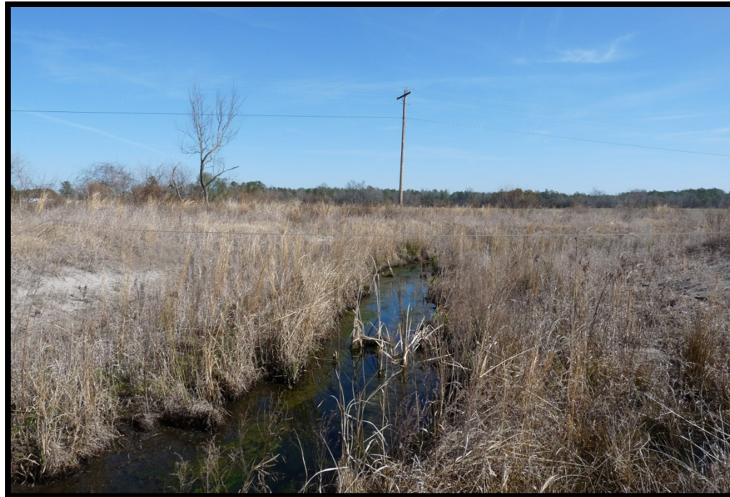
XS 3, Sta. 14+92, Looking Downstream
