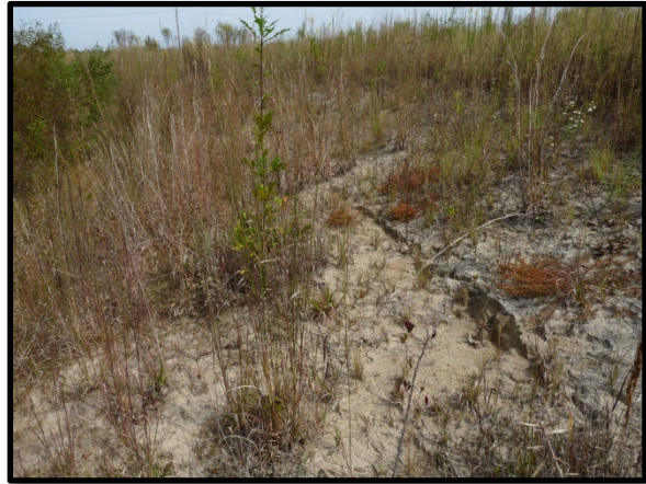
3.18 Minor wash on terrace slope near station 27+50
