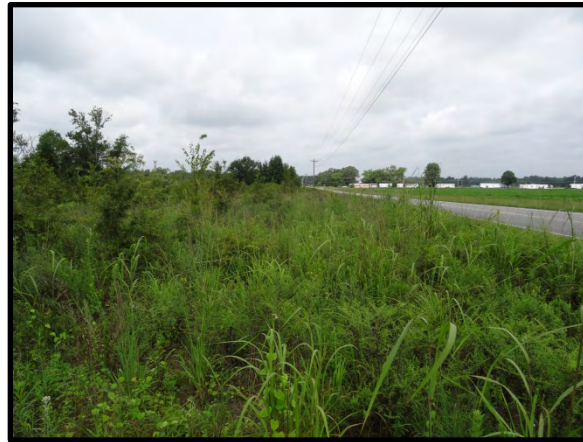
Figure 1.0 Evidence that mowing has ceased underneath power line
