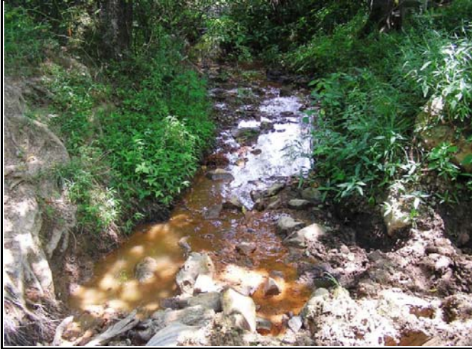
Downstream of culvert outlet
