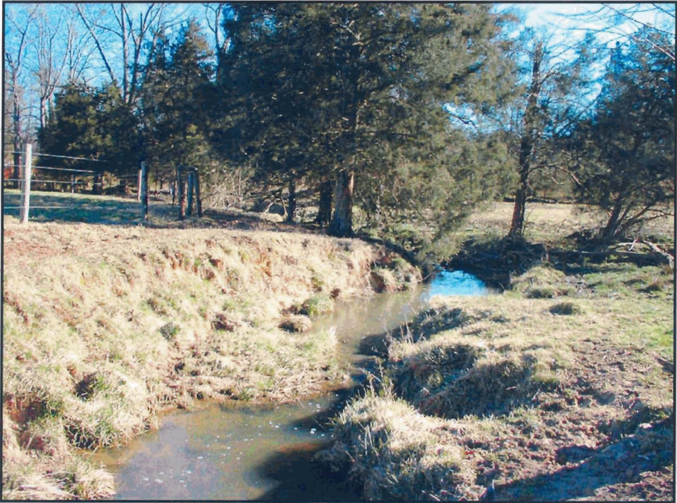
View of Upstream MC looking north (downstream).
