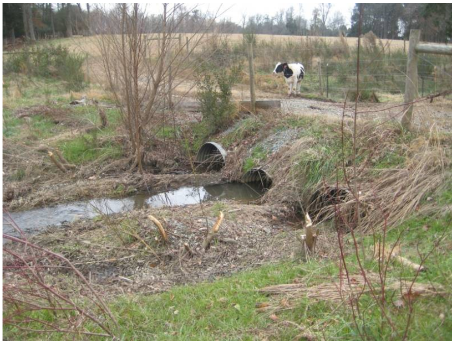
SPA 5B Downstream of Crossing
