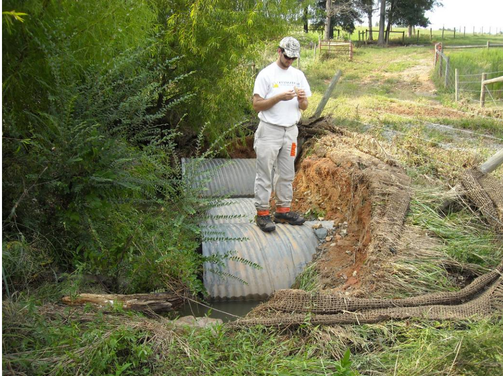
Photo 1. Erosion occurred around culverts during bankfull event in September 2008. Notice on the left the one of many invasive exotic Chinese privet ( Ligustrum sinense ) shrubs observed on site.
