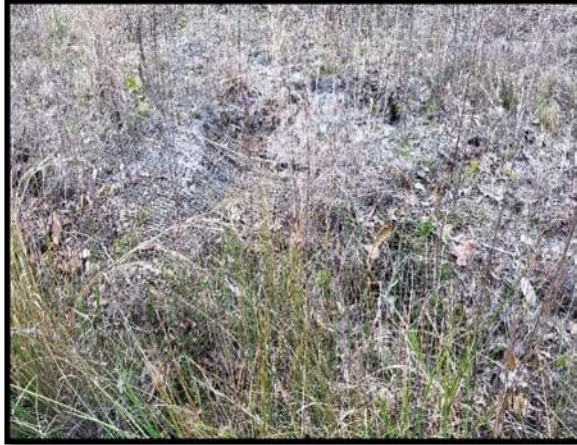
4.13 Minor erosion on right bank at STA 18+50
