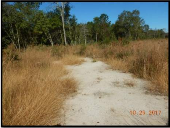
4.10 Bare area near STA 24+00
