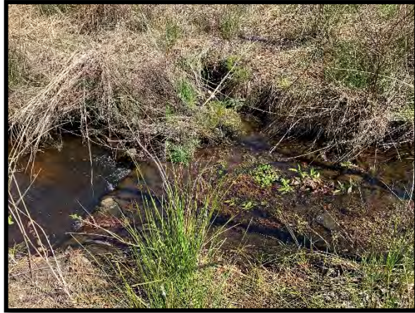
3.12 Moderate erosion near XS 9
