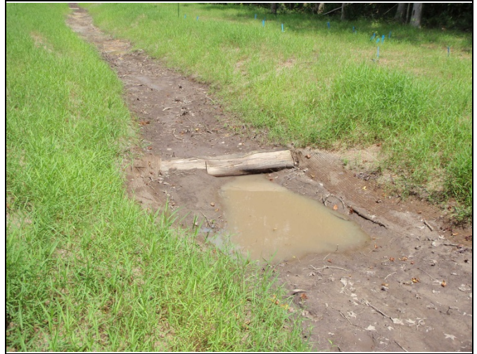
Photo Point 16, UT1a – Station 14+60 (August 13, 2013)
