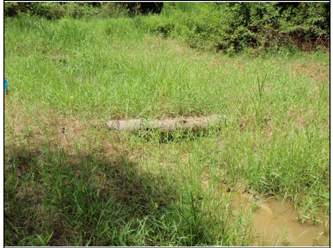
Photo Point 12, UT3 – Station 19+25 (August 13, 2013)
