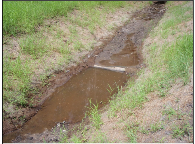
Photo Point 18, UT1a – Station 10+60 (August 13, 2013)
