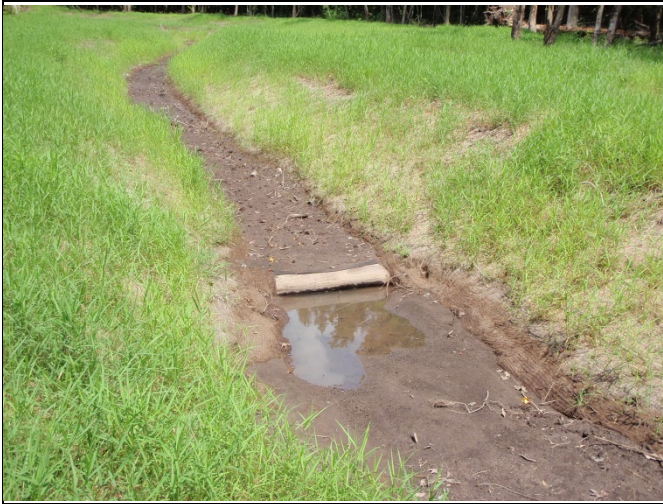
Photo Point 17, UT1a – Station 12+75 (August 13, 2013)
