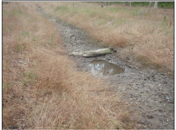
Photo Point 16 – Log Weir
