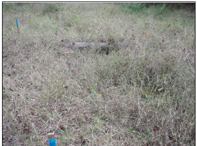
Photo Point 12 – UT3 Log Weir
