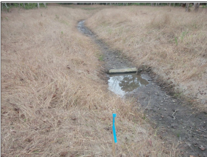
Photo Point 17 – Log Weir
