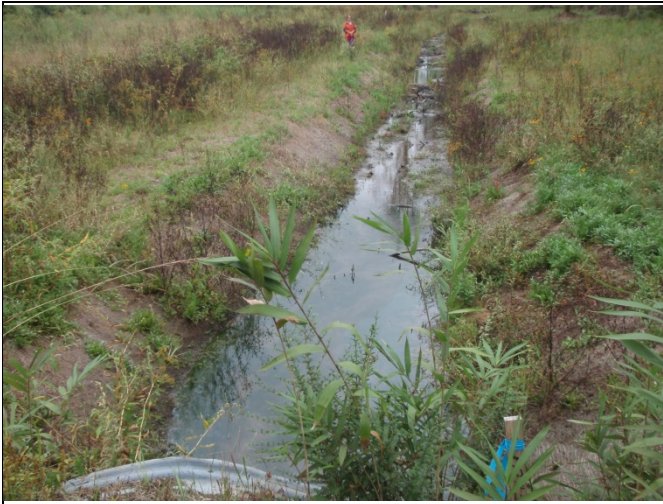
Photo Point 1 – Downstream at Culvert
