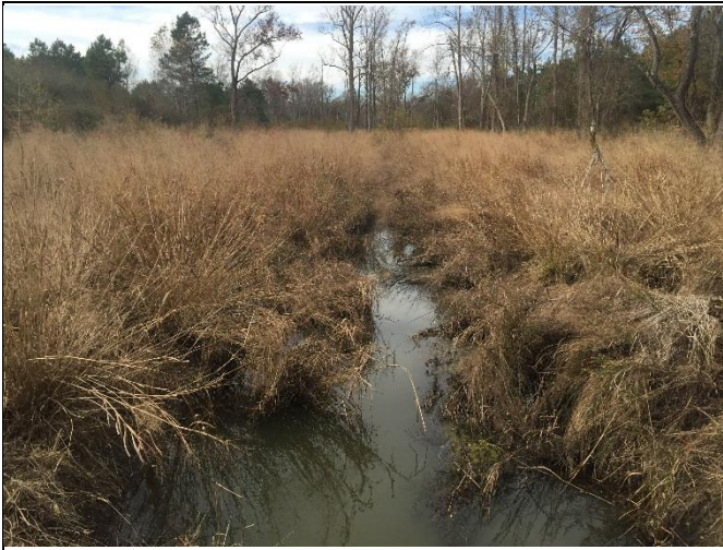
Photo Point 1 – Downstream at Culvert
