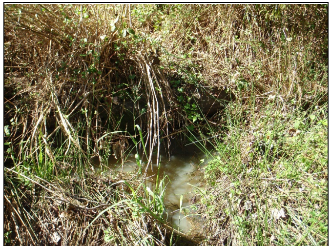
Photo Point 12 – UT3 Log Weir
