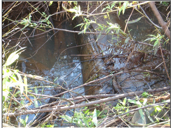
Photo Point 4 – Log Weir/Log Jam
