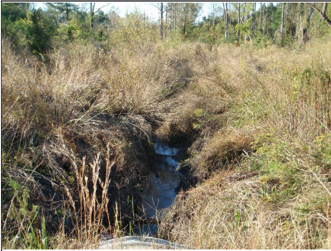
Photo Point 1 – Upstream at Culvert
