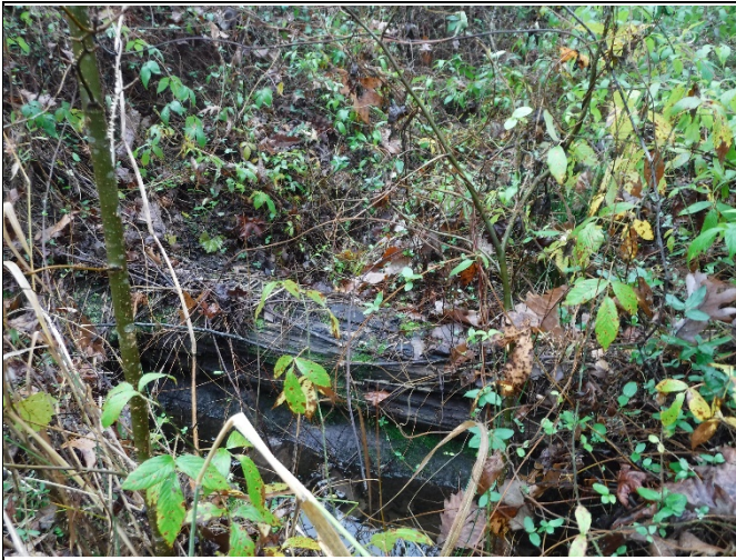
Photo Point 13 – UT3 Log Weir
