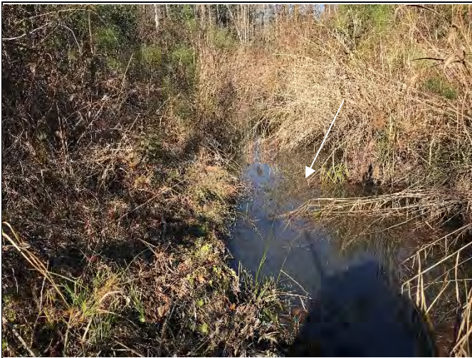
Photo Point 17 – UT1a Log Weir, view upstream
