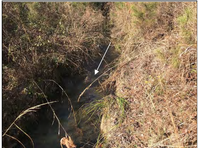
Photo Point 18 – UT1a Log Weir, view upstream
