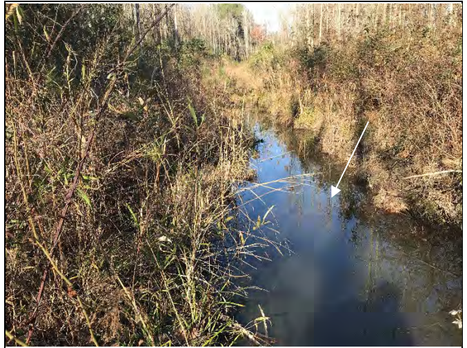
Photo Point 16 – UT1a Log Weir, view upstream
