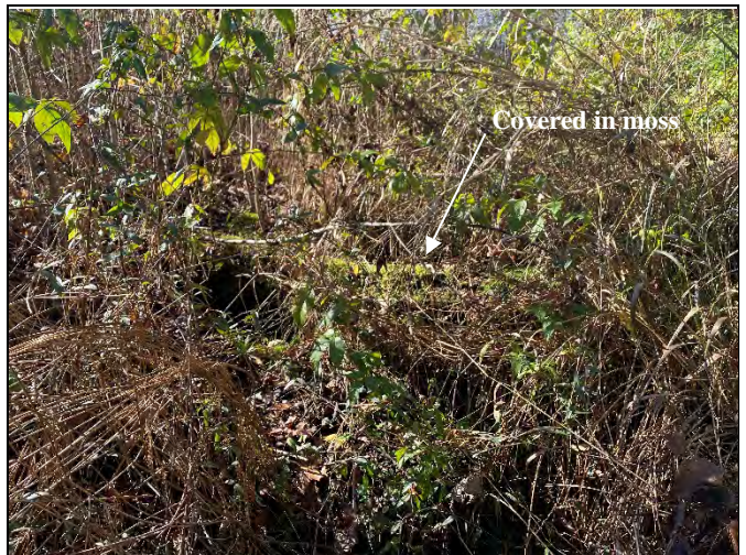
Photo Point 12 – UT3 Log Weir, view upstream
