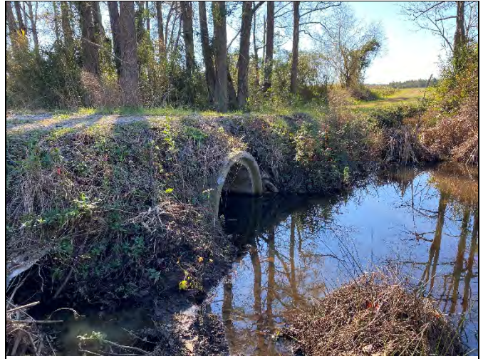
The culvert at the crossing between Reaches UT1b and UT1c
