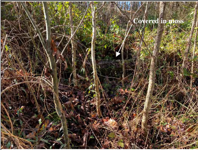
Photo Point 13 – UT3 Log Weir, view upstream
