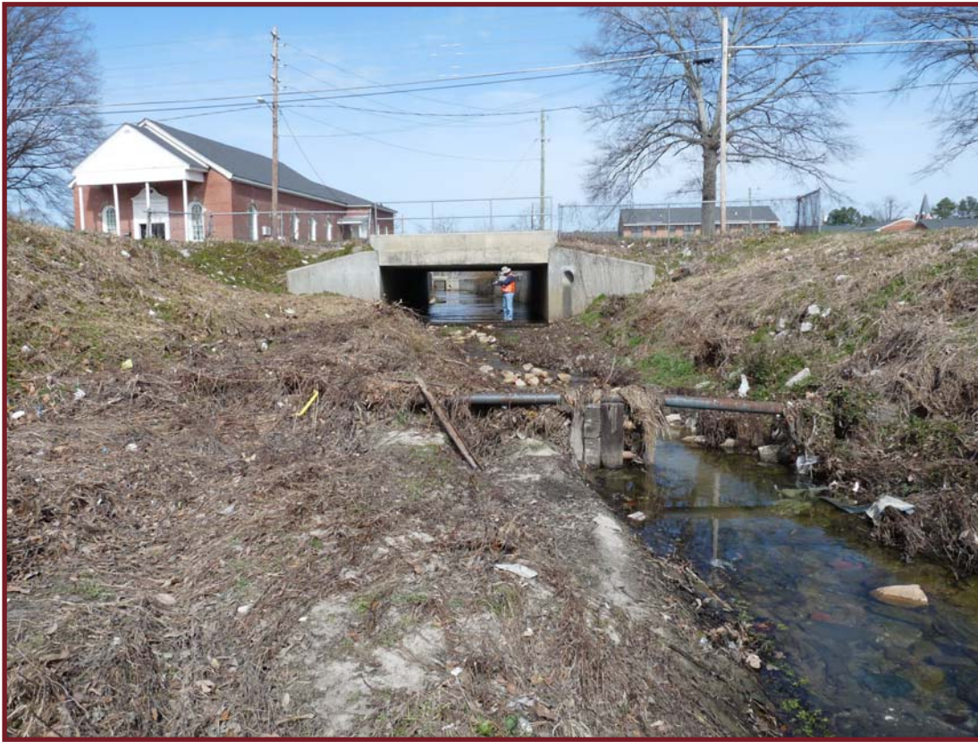
Photo 1 - Sewer service line within channel
