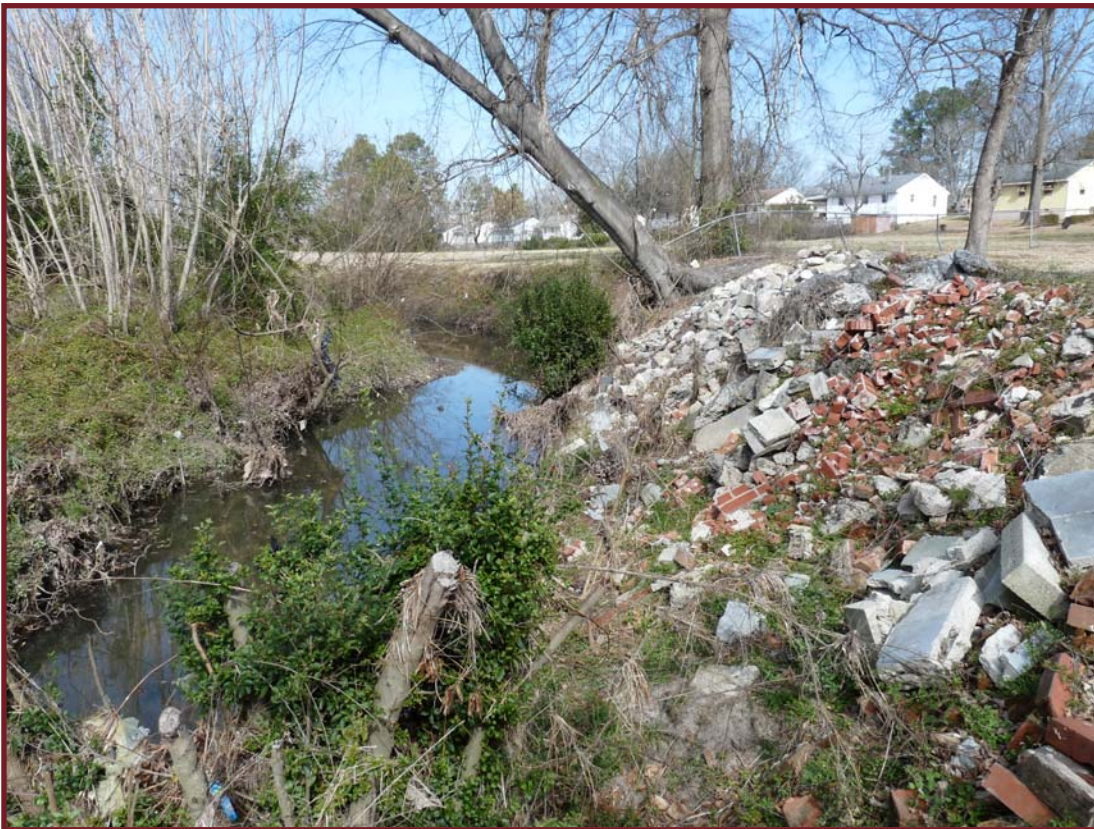
Photo 4 – Eroding banks stabilized with scrap concrete and brick material
