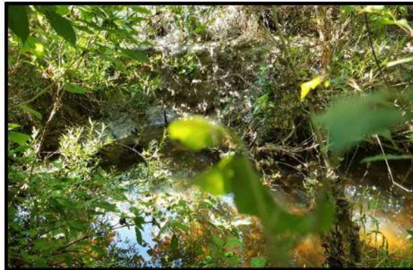
3.14 Moderate Erosion Station 29+25
