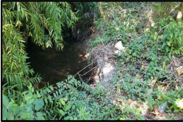
3.12 Moderate Erosion Station 20+60
